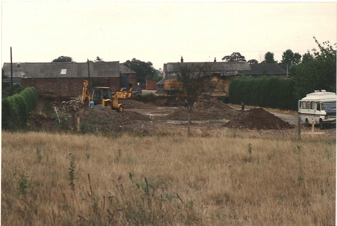
PI. 2 Development plot after removal of vegetation, looking south.
