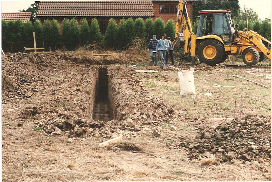
Pl. 3 Development plot during excavation of foundation trenches, looking west.
