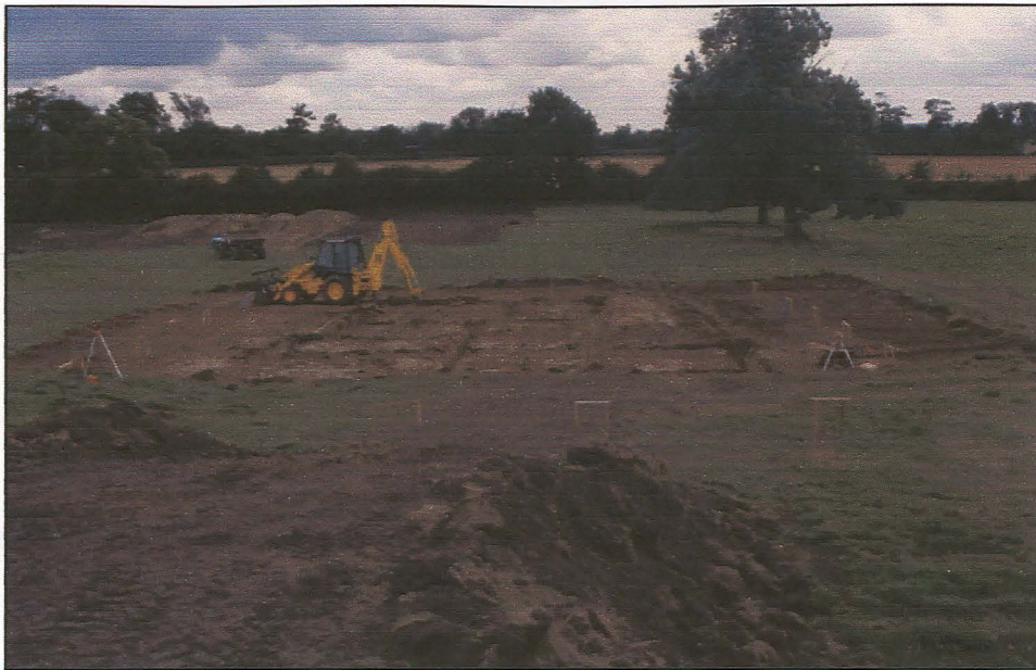
Plot 3 General view looking south west
