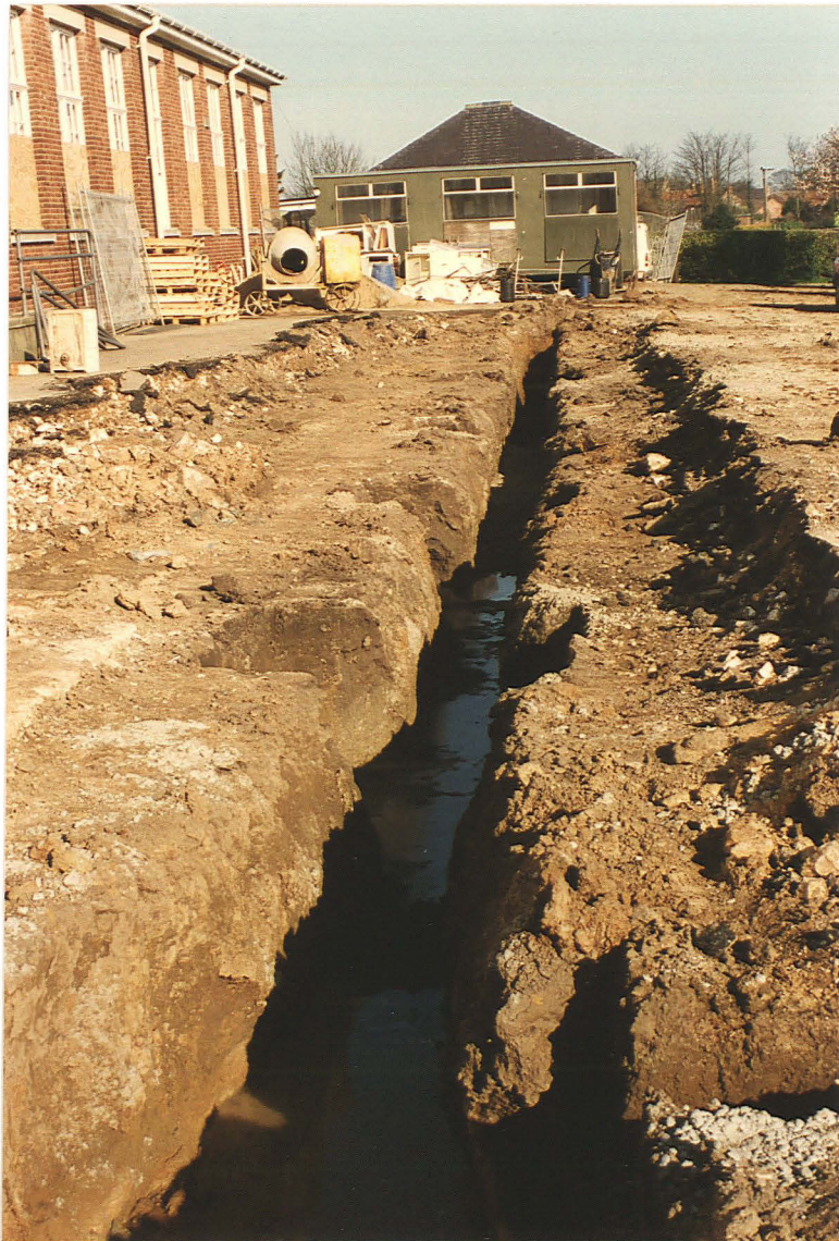
Pl. 6 The western wall trench, after concreting. Looking NW from D7.
