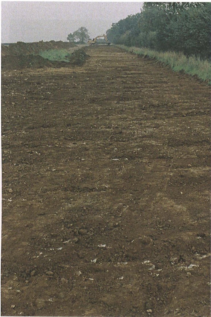
Pl. 5. Machine stripping of easement in excavation area, looking east.
