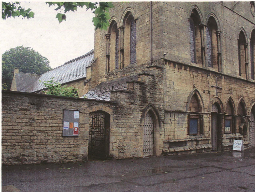
Plate 1 – View of the northwest external corner of the church and the boiler room, looking southeast
