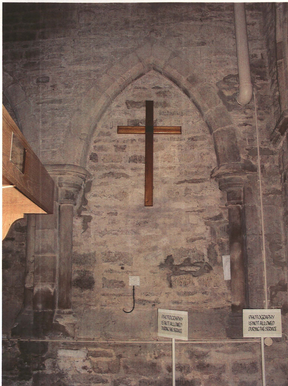
Plate 4 – The blind arcade within the church through which the proposed passage exits. Much of the stonework has been re-cut using a saw and has pronounced tooling marks not typical of medieval work.
