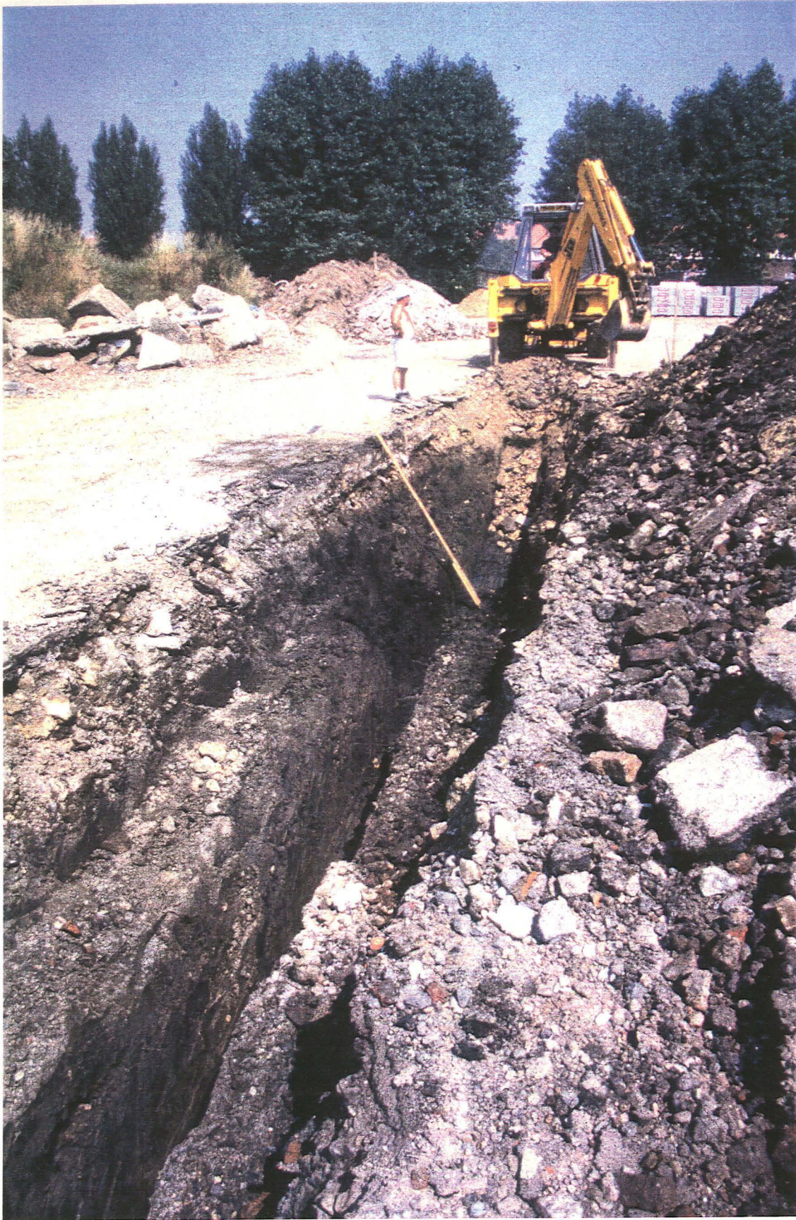
Plate 2. View along Drainage trench, looking North
