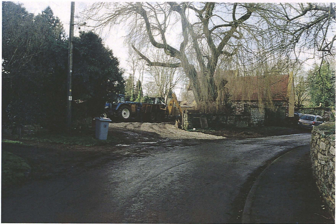
Pl. 1 9 Pond St Harlaxton, general site view looking south-west
