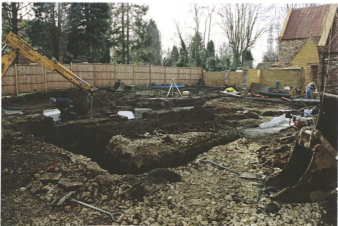
Pl. 2 Excavation of the foundations in progress, looking south-west
