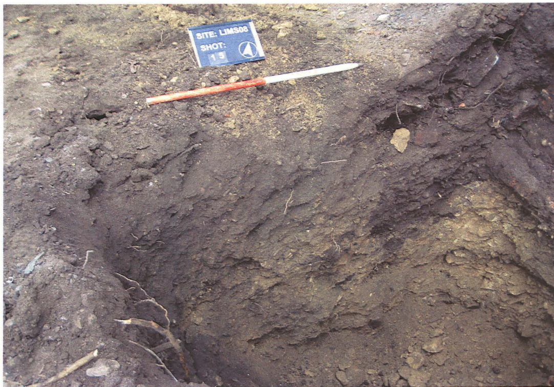
Plate 10 – Section 4: Excavation for underpinning of adjacent building
