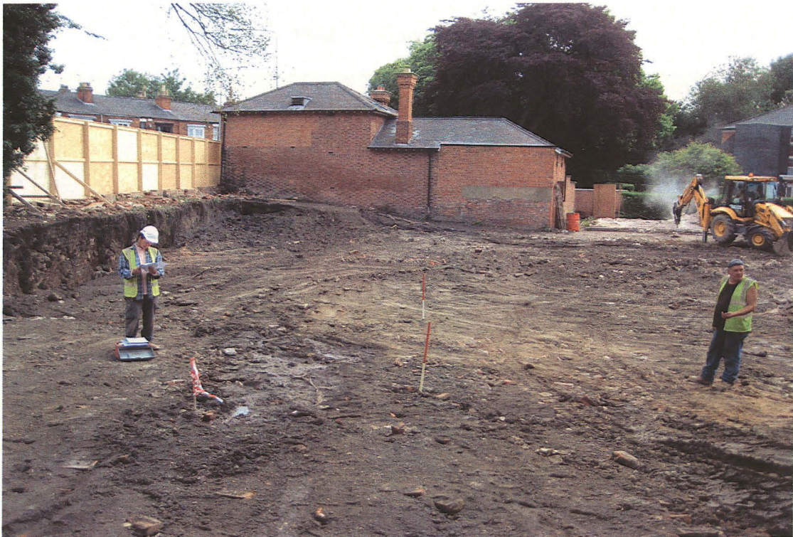
Plate 2 – General view of site
