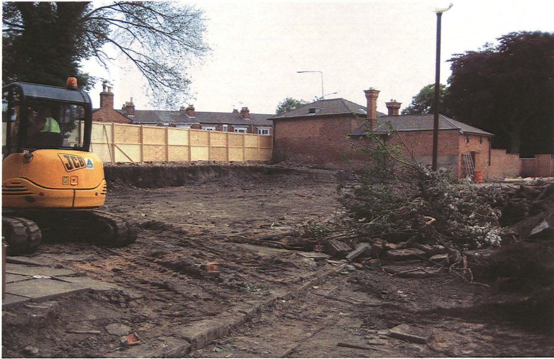
Plate 1 – General view of site
