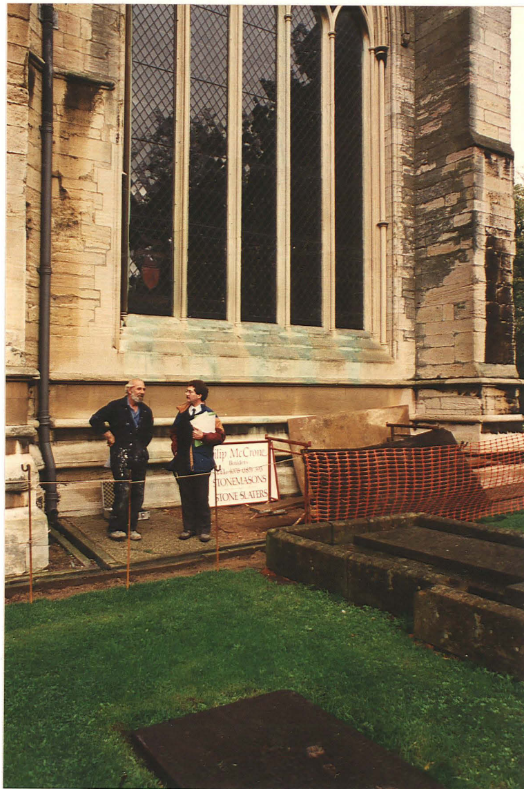
Pl. 9 South aisle W wall showing concrete apron between buttresses.
