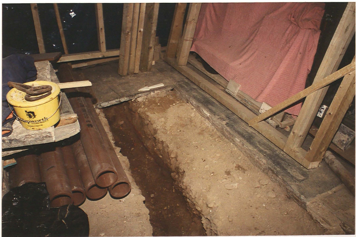
Pl. 8 Foundation trench along S wall of store showing edge of brick vault
