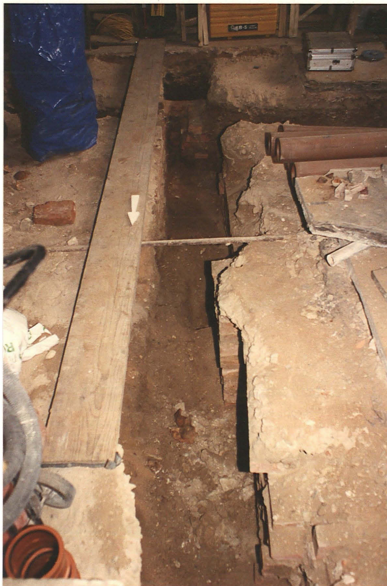
Pl. 7 Foundation trench for office E wall, looking S, showing edge of double vault and vault beyond
