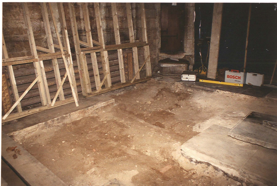
Pl. 2 W end of area after removal of floor makeup, showing traces of brick cross walls, in area of proposed toilets
