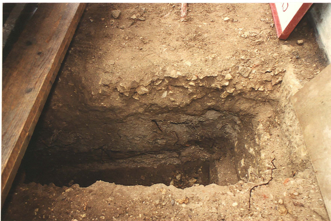
Pl. 10 Sewer trench perpendicular to aisle W wall, showing off-set footings
