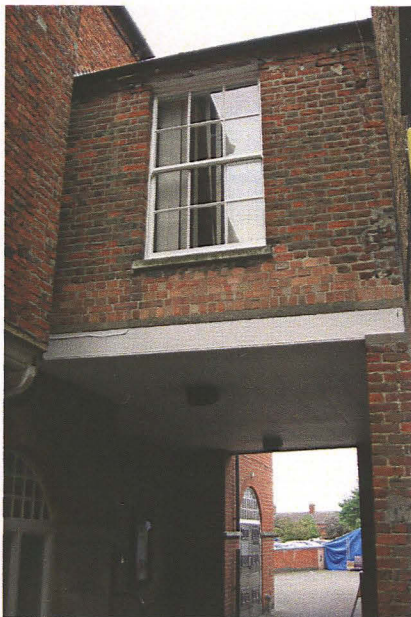
Pl. 27 Retiring room, looking east, note the rebuilt area below the window.
