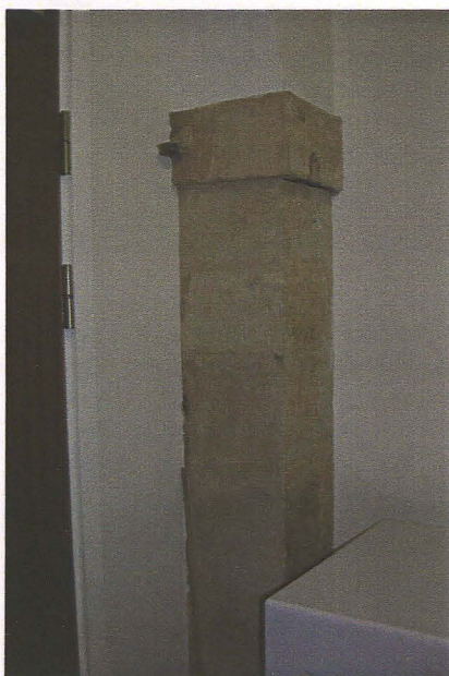
Pl. 7 Main office, example of stone pillar with pintle for hanging gate.
