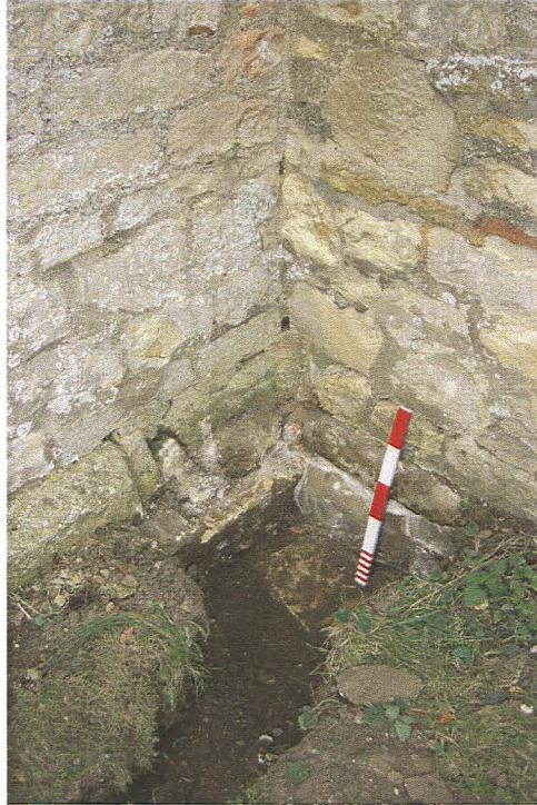
Pl. 7 Junction of south aisle and chancel foundations, looking north, scale 0.50m
