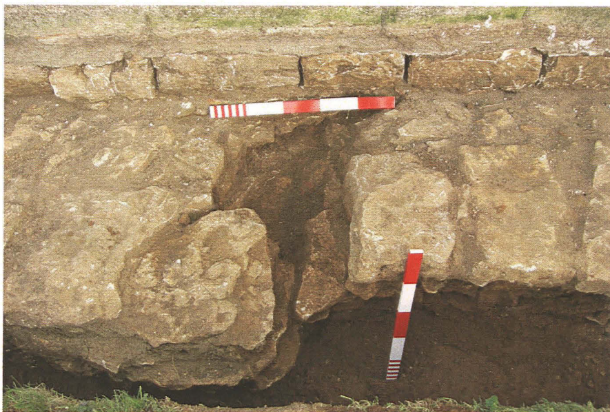
Pl. 22 Tower west foundations, disturbed area near north-west angle, looking east
