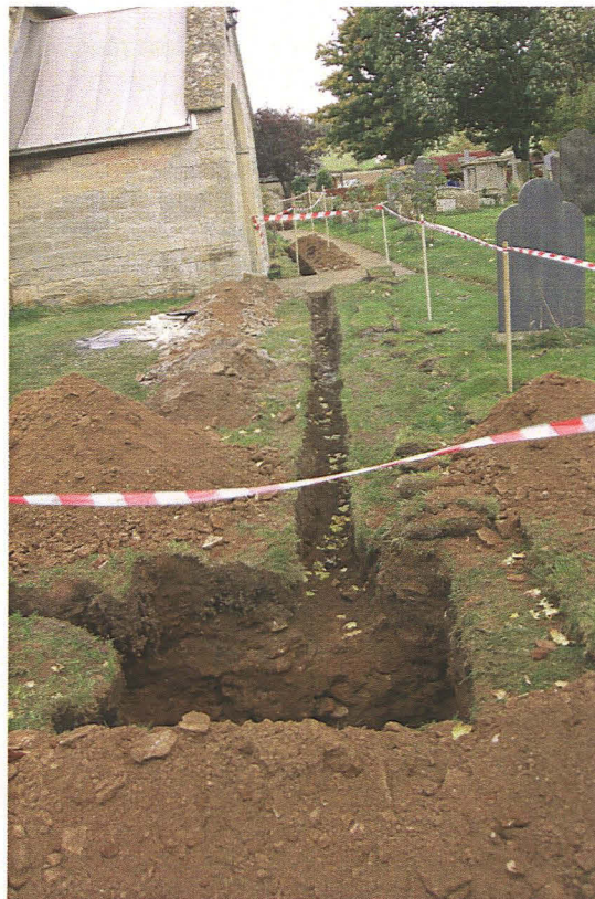
Pl. 6 Drain trench along south side of the church , looking east
