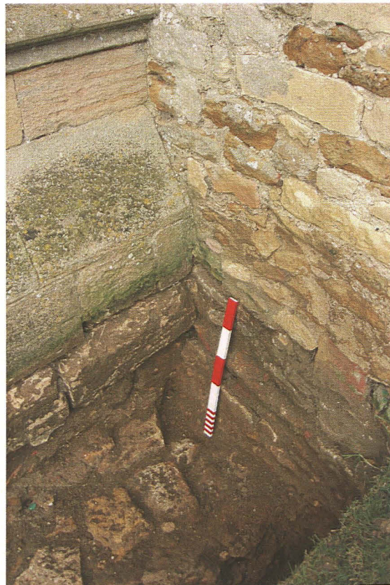
Pl. 26 Junction of tower and south aisle foundations, scale 0.50m
