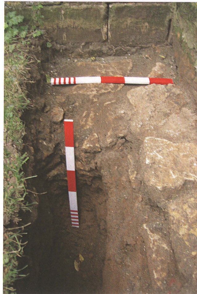
Pl. 18 Junction of tower and north aisle foundations
