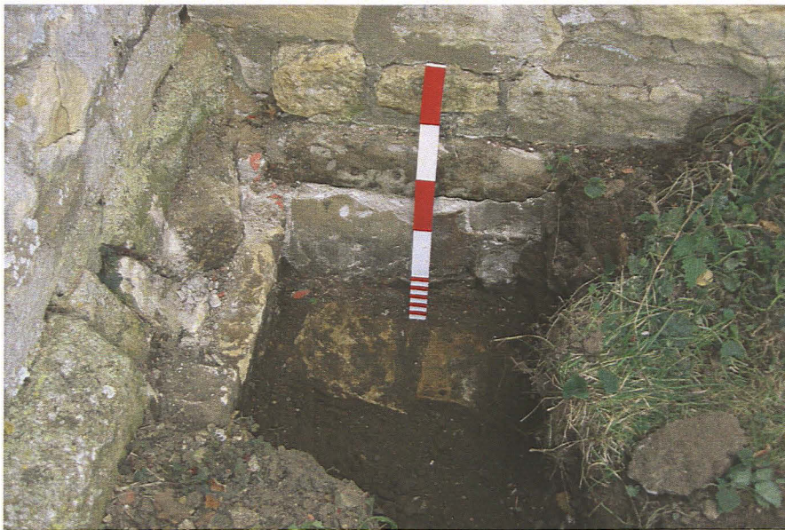
Pl. 8 South aisle and chancel foundations detail , looking north, scale 0.50m
