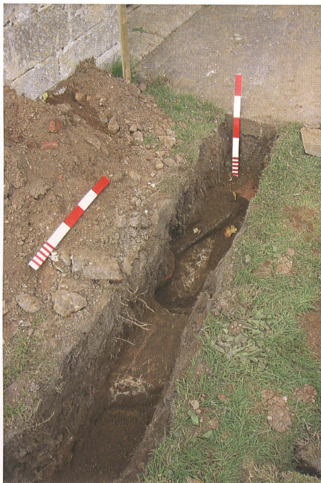
Pl. 13 Porch foundations, south-west corner, looking north-east
