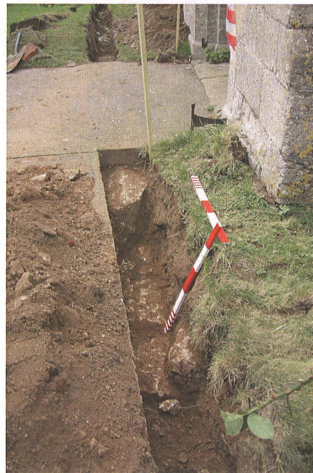
Pl. 14 Porch foundations, south-east corner, looking north-west
