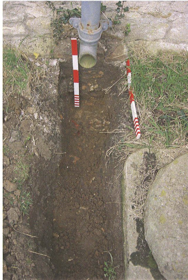
Pl. 10 South aisle foundations, scales 0.50m
