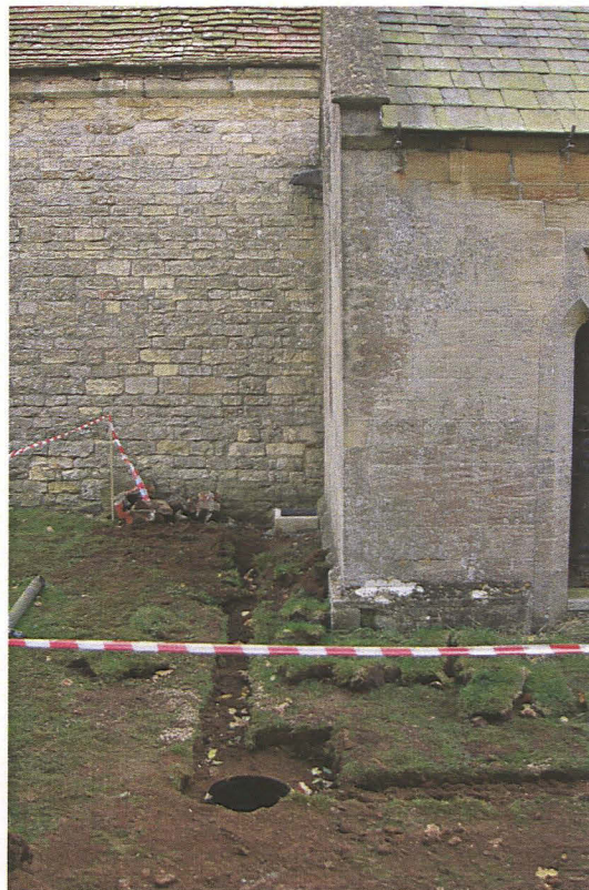
Pl. 2 Drain trench along east side of vestry, looking south
