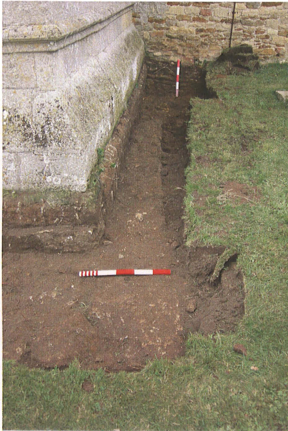
Pl. 23 Tower south foundations, looking east
