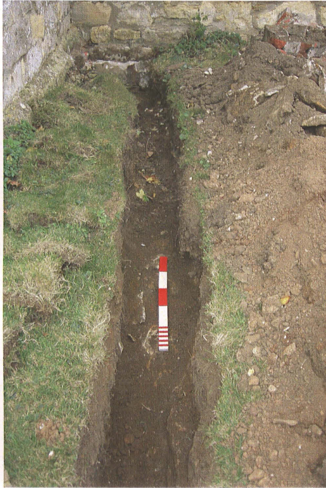
Pl. 11 Drain run on south aisle east wall, scale 0.50m
