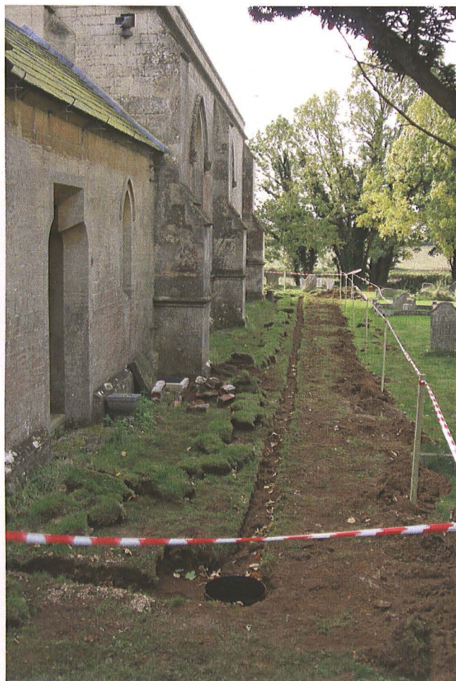
Pl. 3 Drain trench along north side of church looking west
