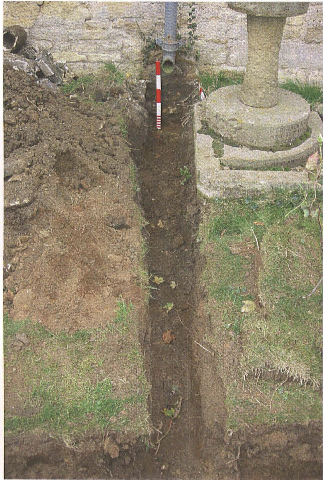
Pl. 9 Drain run on south wall of south aisle
