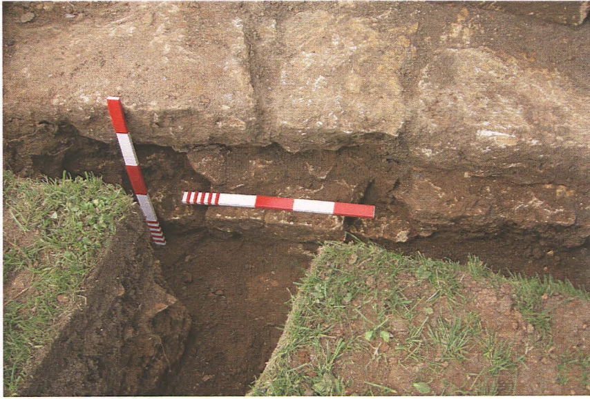
Pl. 25 Tower south foundations, looking west, scale 0.50m
