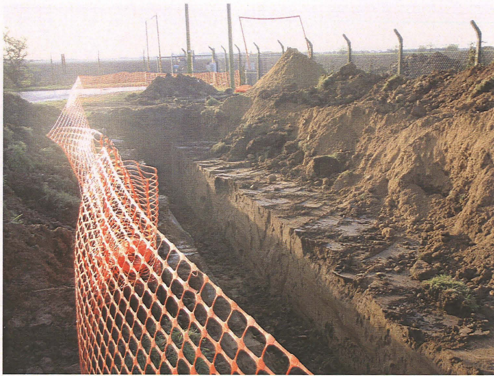
Pl. 7 Pits 11 and 12 (looking north).
