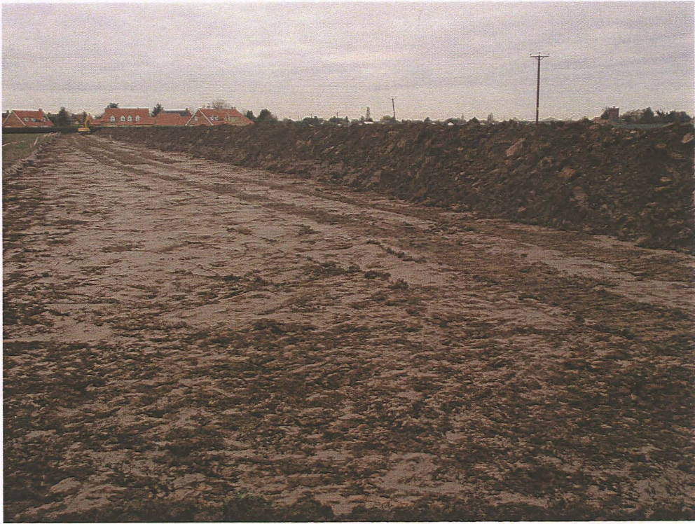
PI. 1 The pipeline easement west of Wythes Lane (looking west).
