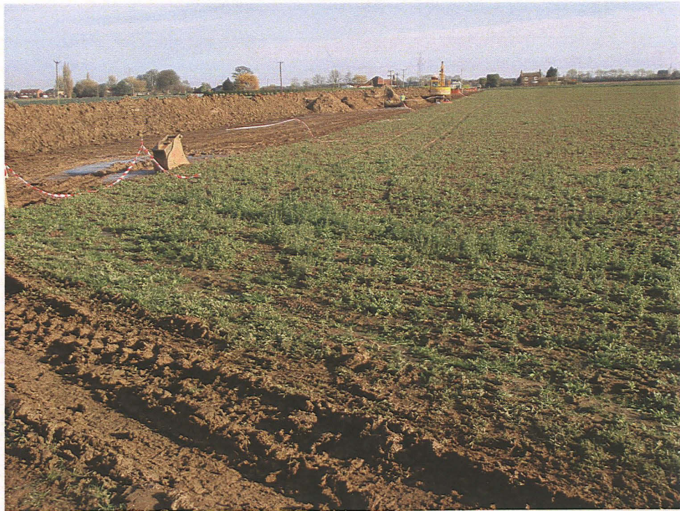
PI. 2 The pipeline easement east of Wythes Lane (looking west).
