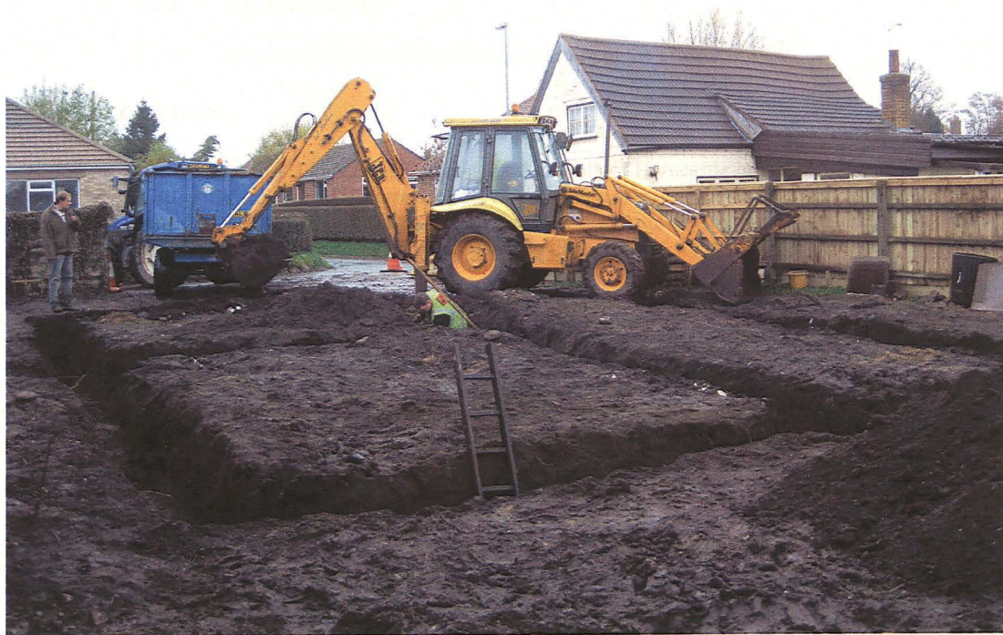
Plate 4. Work in progress looking northeast
