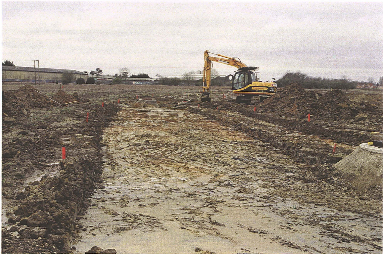
Pl. 3 Field 3. Stripping of the access road, looking south-west.
