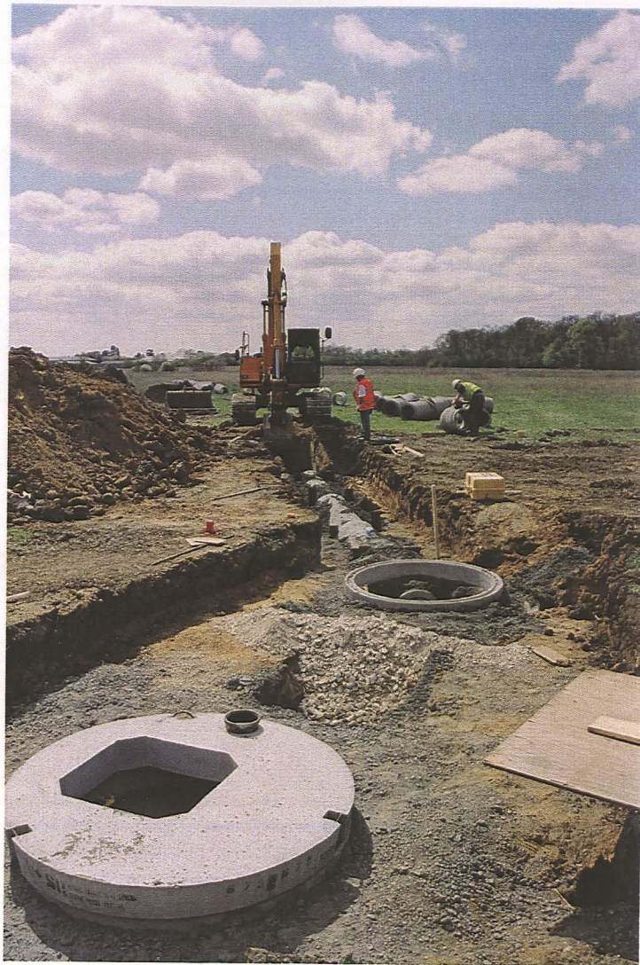
Pl. 1 Field 2 service trench. Note the close proximity of connection points.
