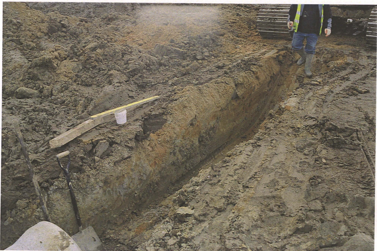
Pl. 2 Field 3 service trench. Note how the smearing of the trench sides makes identification of any archaeology impossible.
