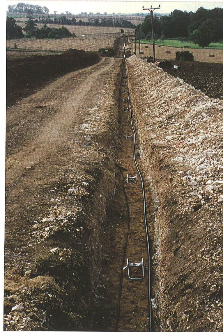
Pl. 1 North end of cable trench at junction with the road from Thorganby. Shows ducting under the road, the sand bedding and the two cables in position.
