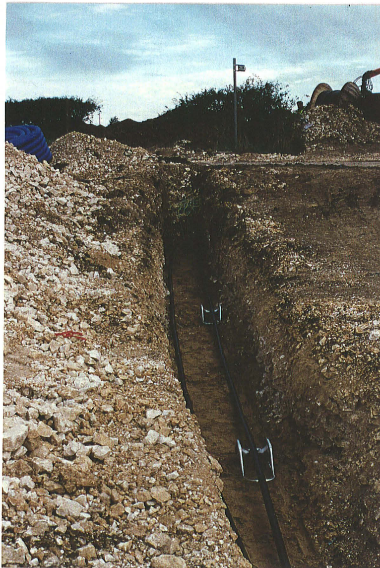
Pl. 1 North end of cable trench at junction with the road from Thorganby. Shows ducting under the road, the sand bedding and the two cables in position.
