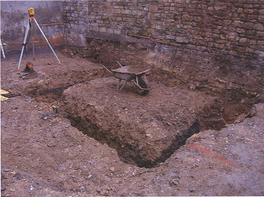
Plate 3: The foundation trenches during excavation
