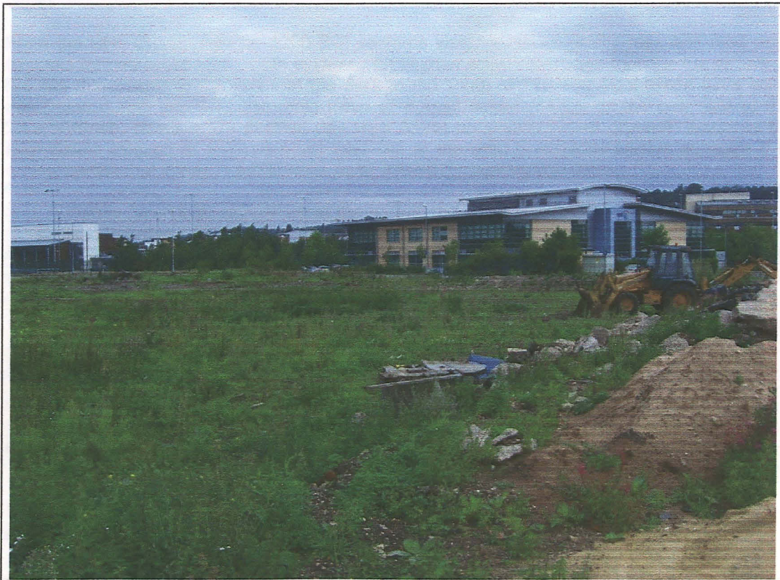
Plate 1: General view of the site looking north.
