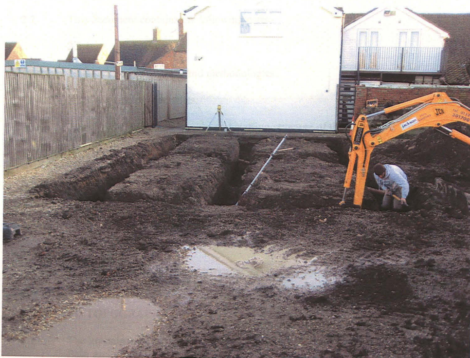
Plate 5. Completed footings looking southeast
