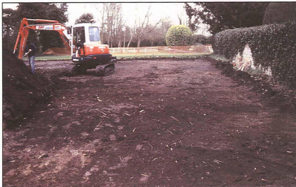
Plate 2: General view of the topsoil strip looking west
