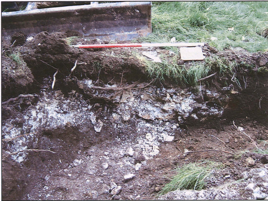
Plate 5: Drainage trench showing foundation (008) and foundation (110) at the left of the photograph, looking west.
