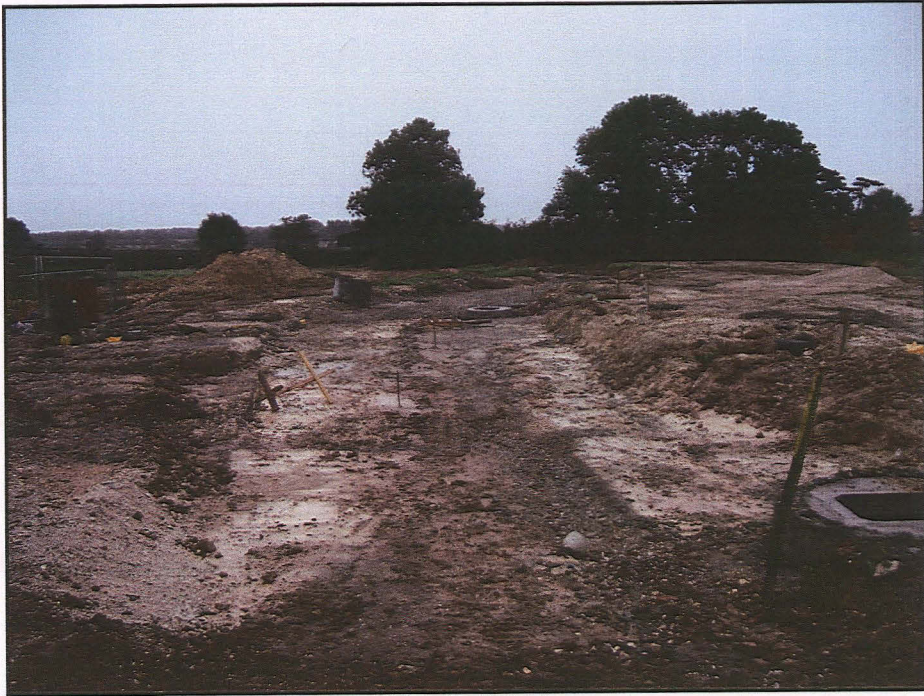
Plate 3: General view of the site looking north
