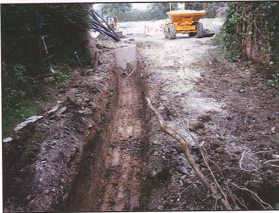
Plate 8: General view of drainage trench along access road looking north
