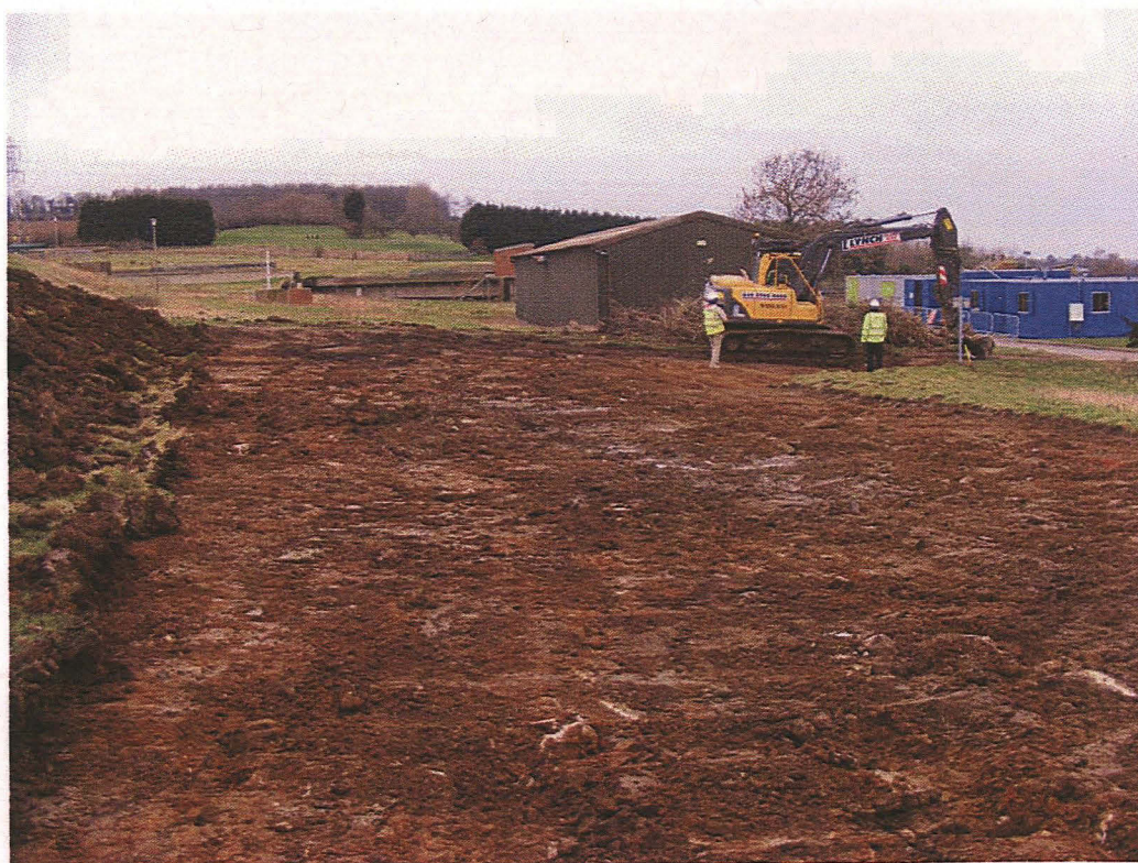
Plate 8: The pipeline route during groundworks
