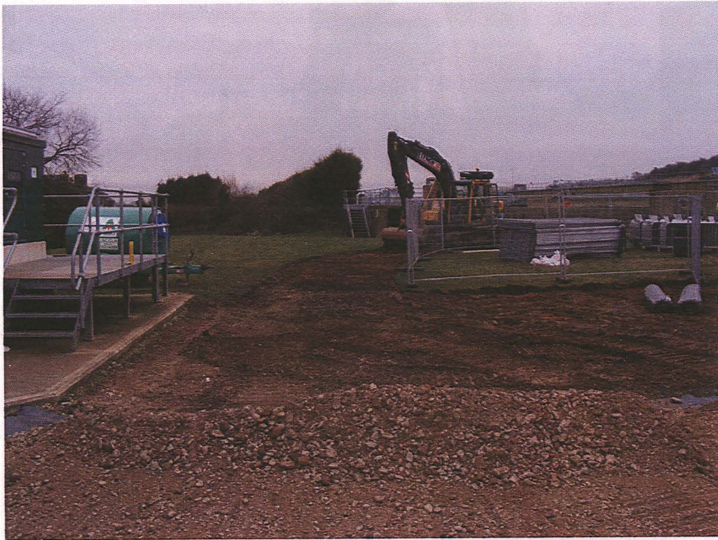
Plate 3: The temporary storage area during groundworks
