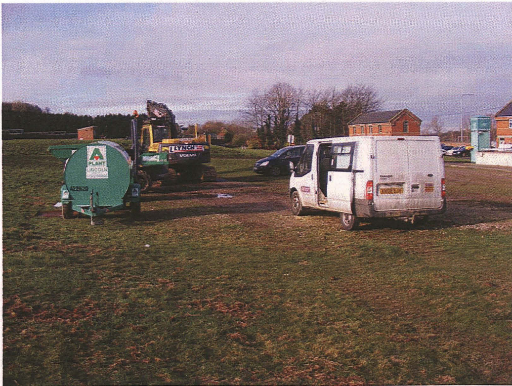
Plate 2: the area of temporary storage at the start of groundworks
