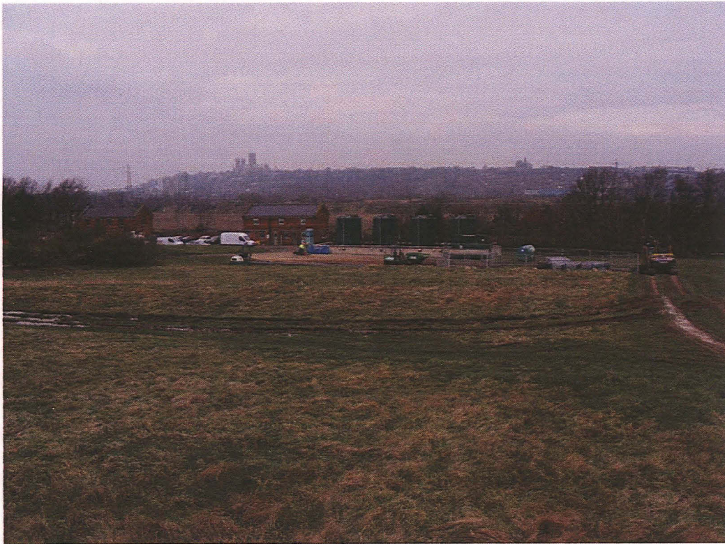
Plate 1: A general view of Canwick sewage treatment works
