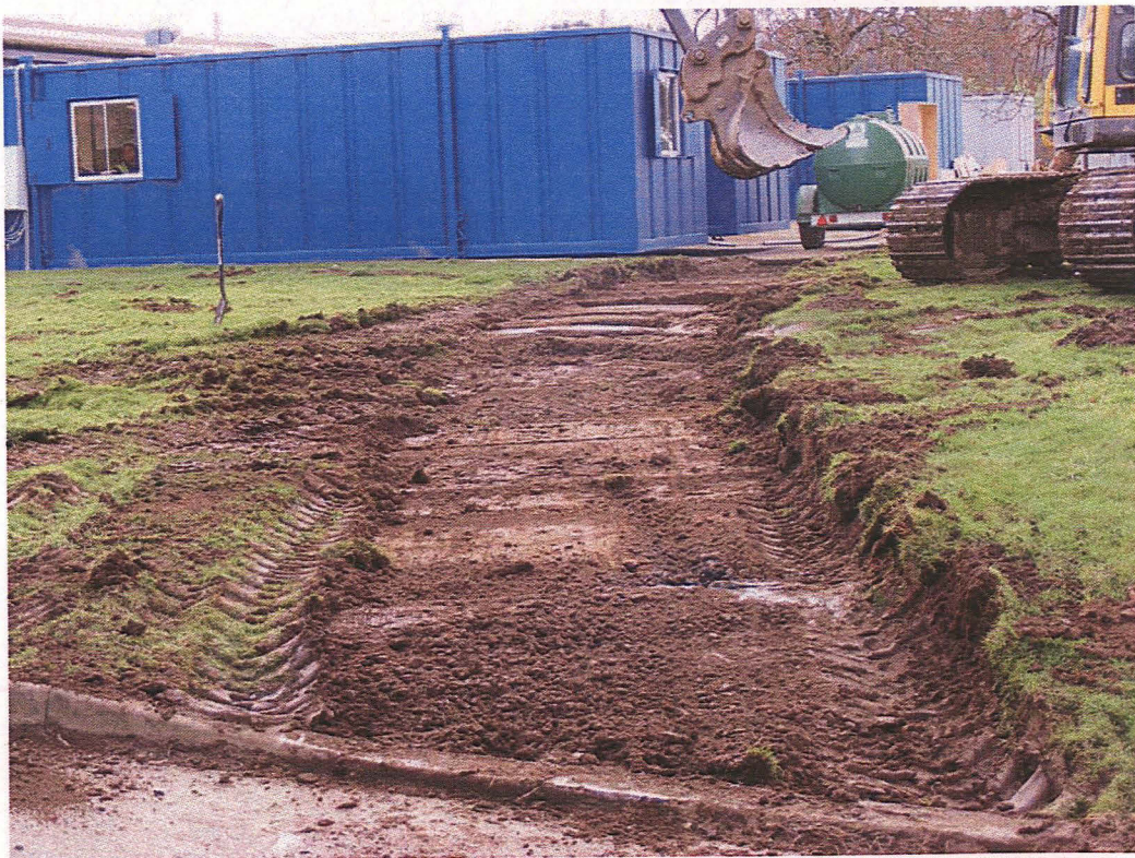
Plate 6: The temporary footpaths during groundworks
