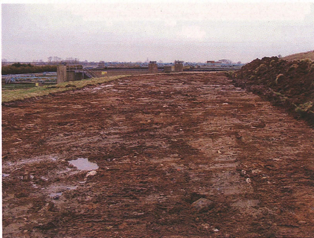
Plate 7: The eastern terminus of the pipeline route during groundworks
