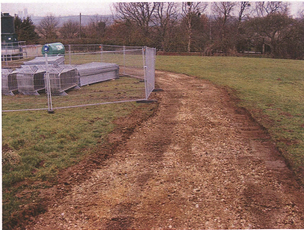
Plate 4: The temporary access road during groundworks
