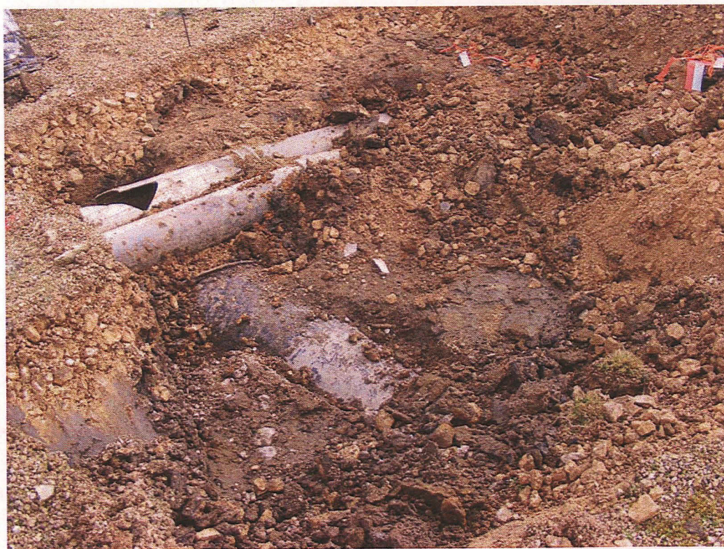
Plate 10: The test pit, western terminus of the pipeline route
