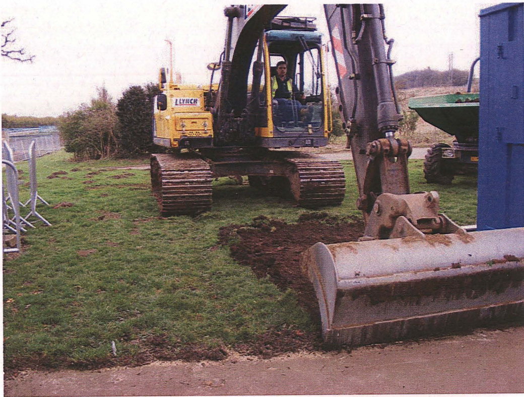
Plate 5: The temporary footpaths at the start of groundworks
