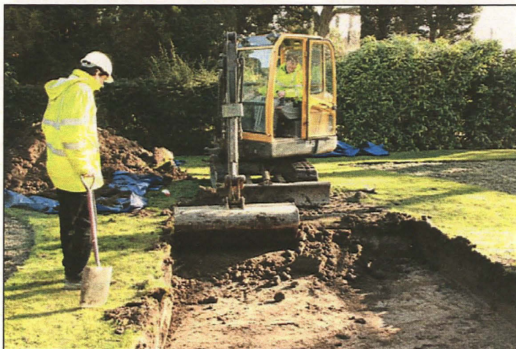
Plate 14. Trench 5: work in progress opening trench, looking north-east.
