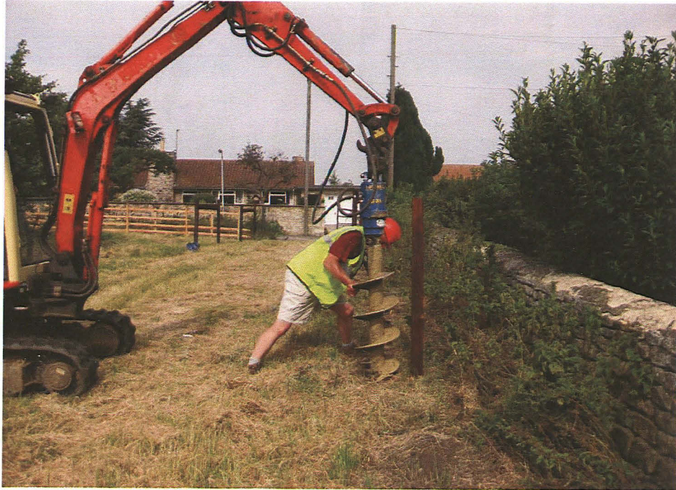
Plate 1 – Drilling of Borehole 1, looking west
