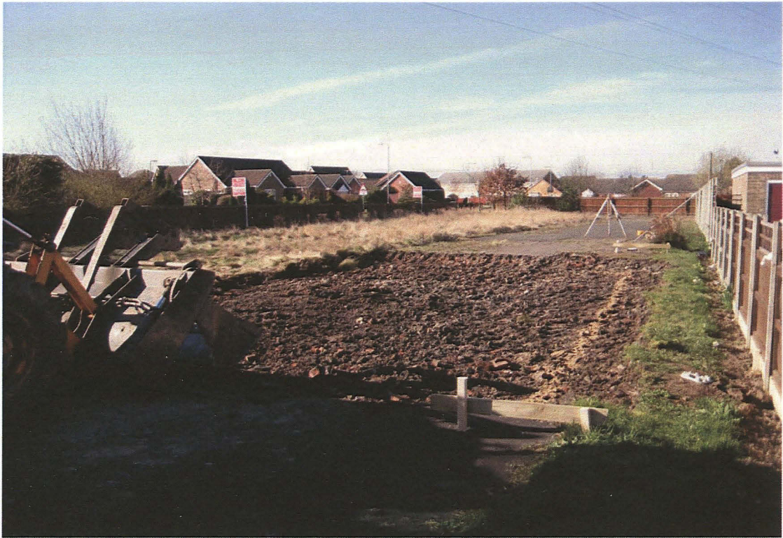
Plate 1 – General view of site
