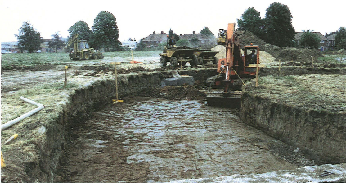
Excavation of the roundabout cutting, looking south: the dark stain in the right hand corner is the backfill of Grubenhäus 1
