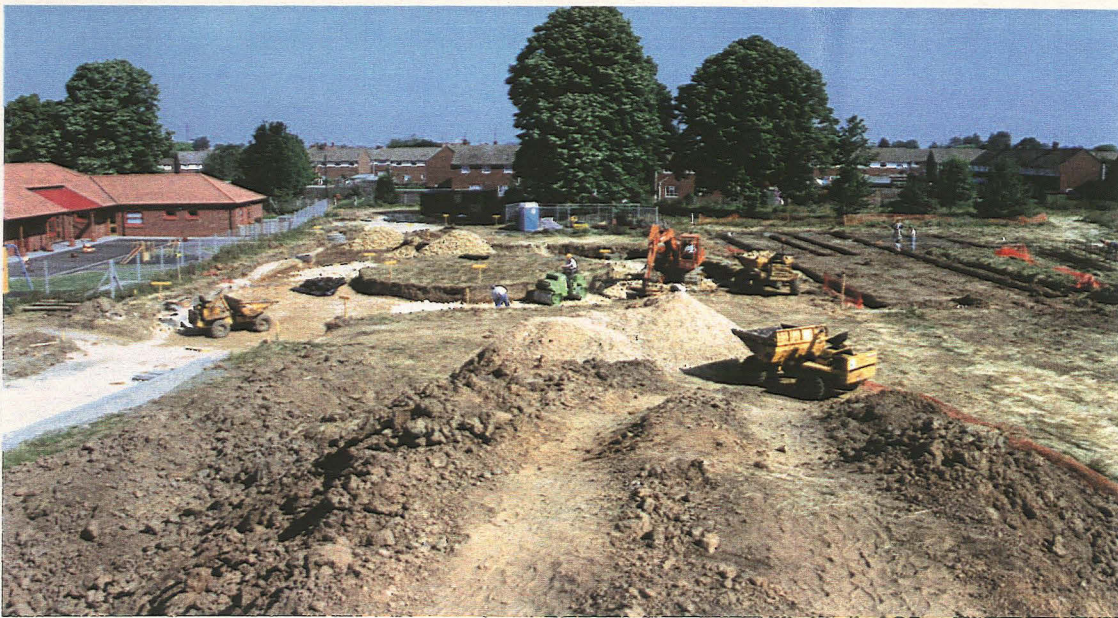
General view of site during earth-stripping, looking north
