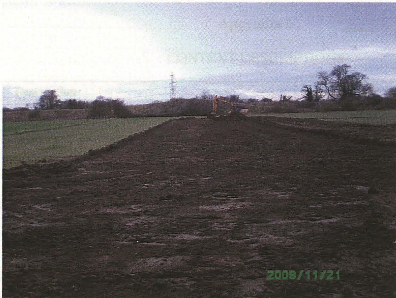
Plate 3. Machining area of poultry units looking west
