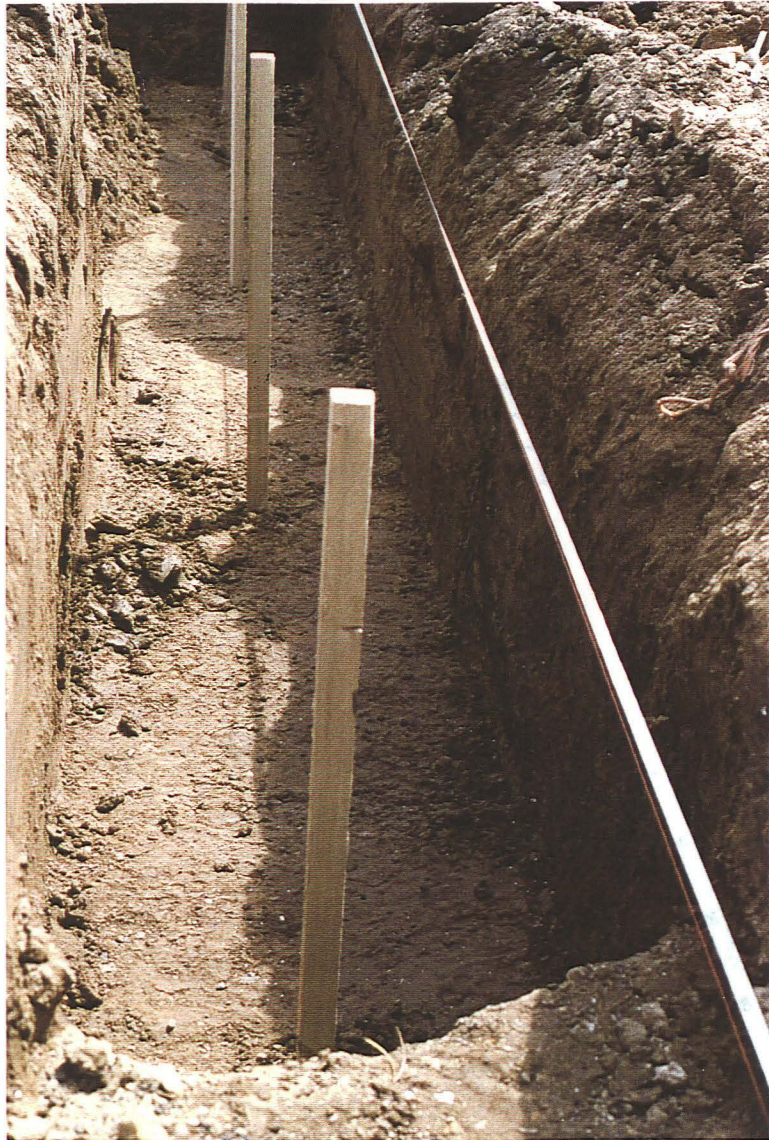
Pl. 21 The southern part of the western trench, with the modern drain in the immediate foreground and the dark fills of 33 behind. (Looking west).
