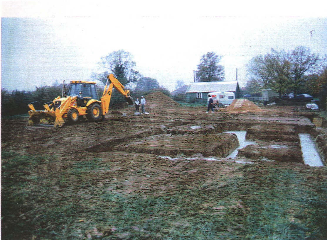
P1. General view of trenched plot following concrete pouring, looking north-west
