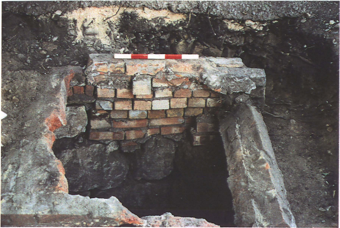
Pl. 3. NE infill repair 23 to wall 22/30 (block 25 in 22 to left); from SW.
