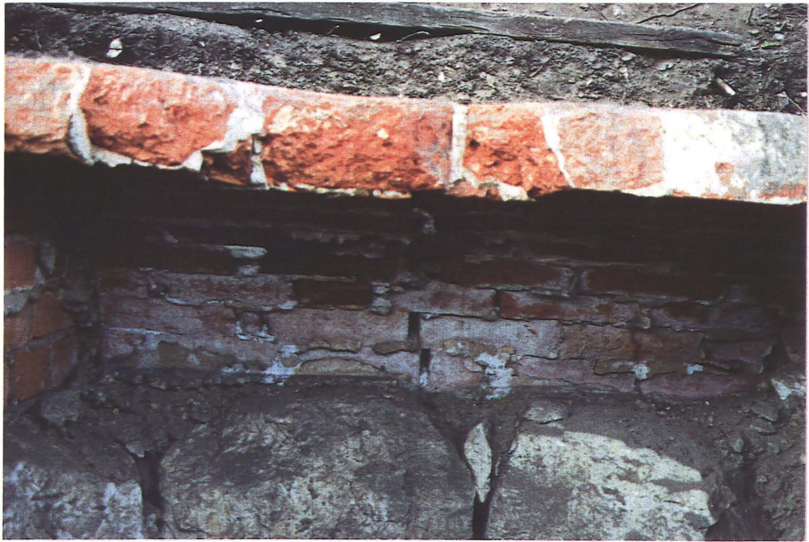
Pl. 11. Broken vaulting intrados 12; mortared springing from truncated stone lining. From SE.
