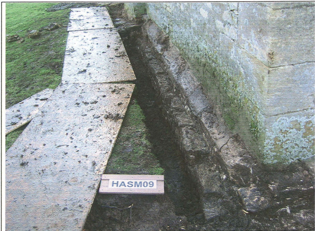
Plate III: General view of excavations at the base of the north tower wall showing the previously buried chamfered string course & projecting stone foundations [005]. Foundation [004] is visible at the very top of the photograph (looking east).
