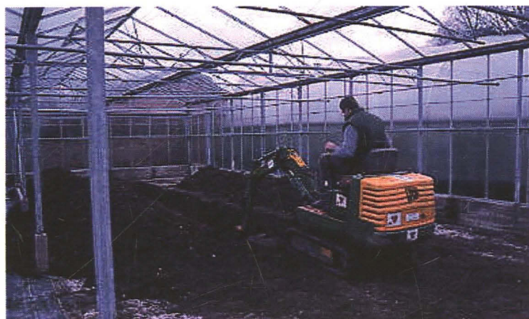
Plate 1: Opening trench 4 with the 1.5T mini-digger.
