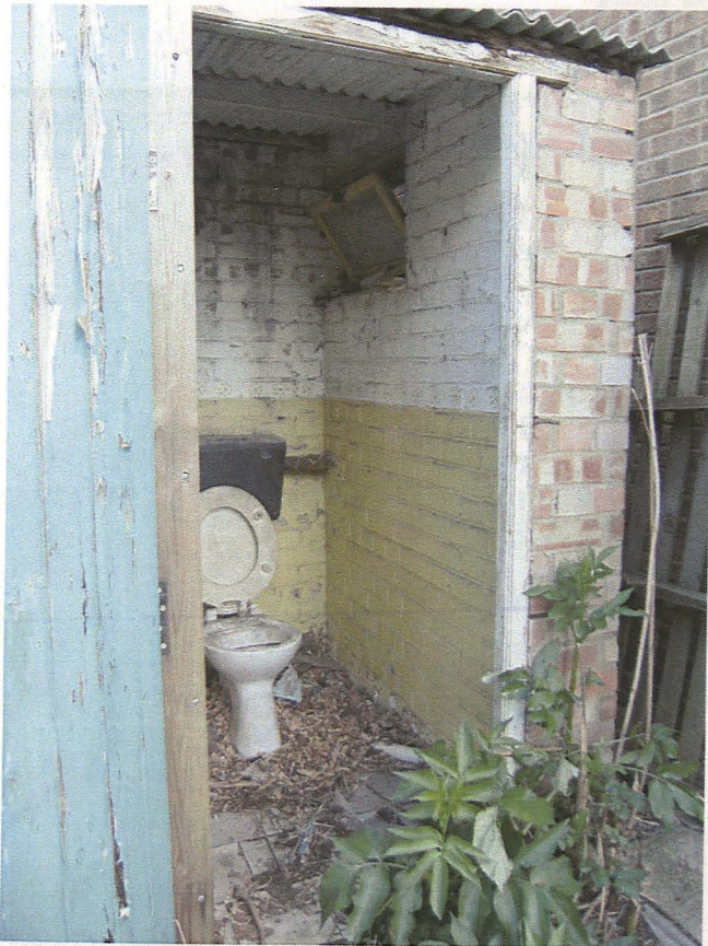
Plate 63 Interior of Room 3a, looking southeast
