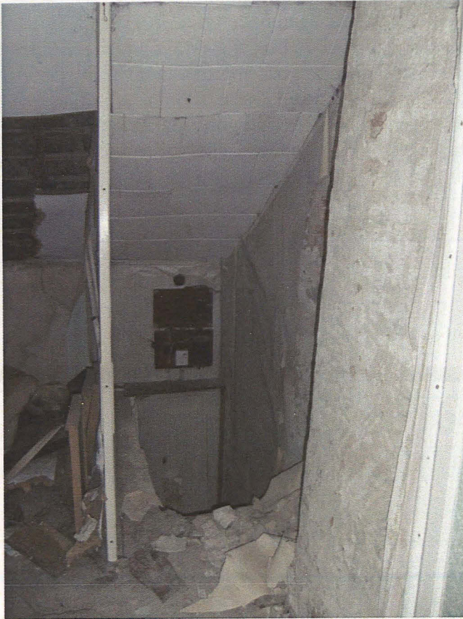
Plate 33 Interior of Room 1b, looking east towards staircase
