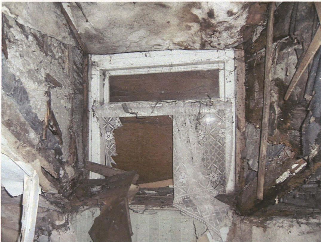
Plate 40 Interior of Room 1b, dormer window, looking east
