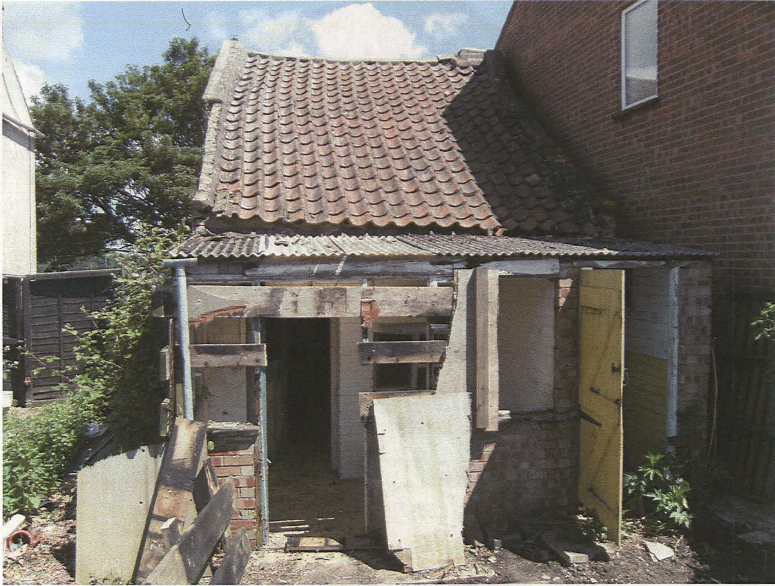
Plate 19 West external elevation of cottage, looking east
