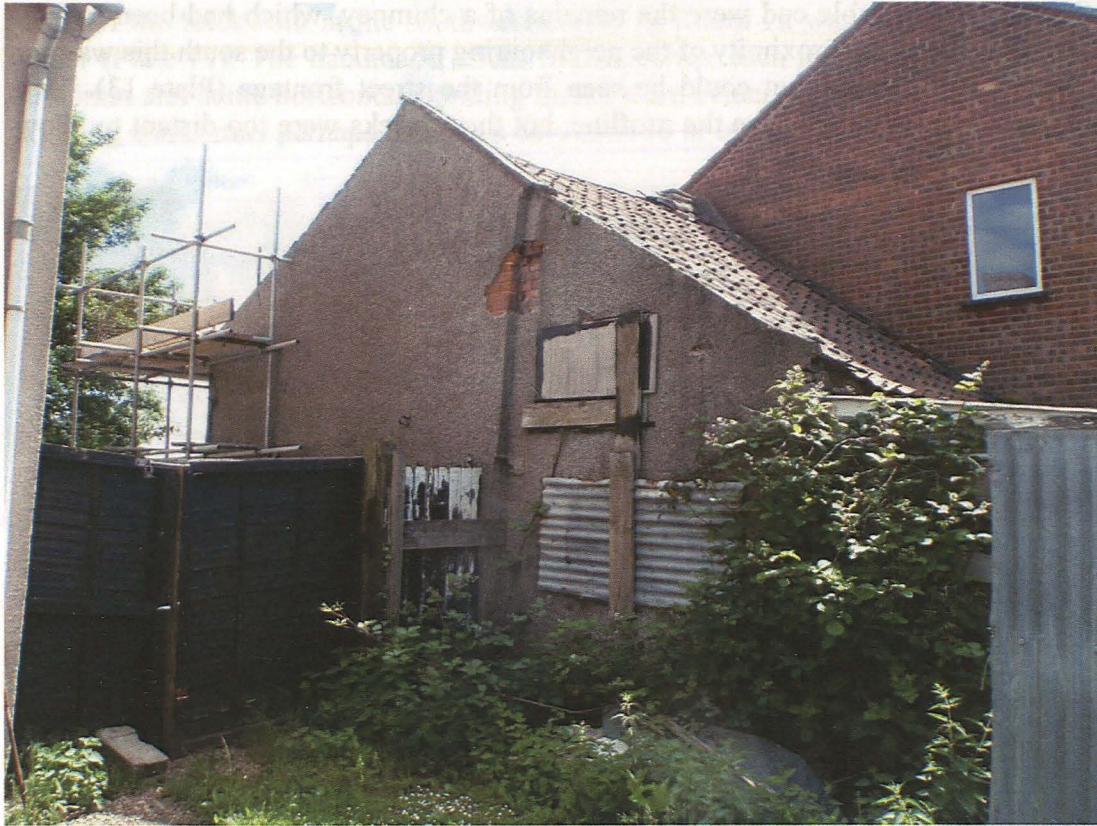
Plate 15 North gable end viewed from neighbouring garden, looking southeast
