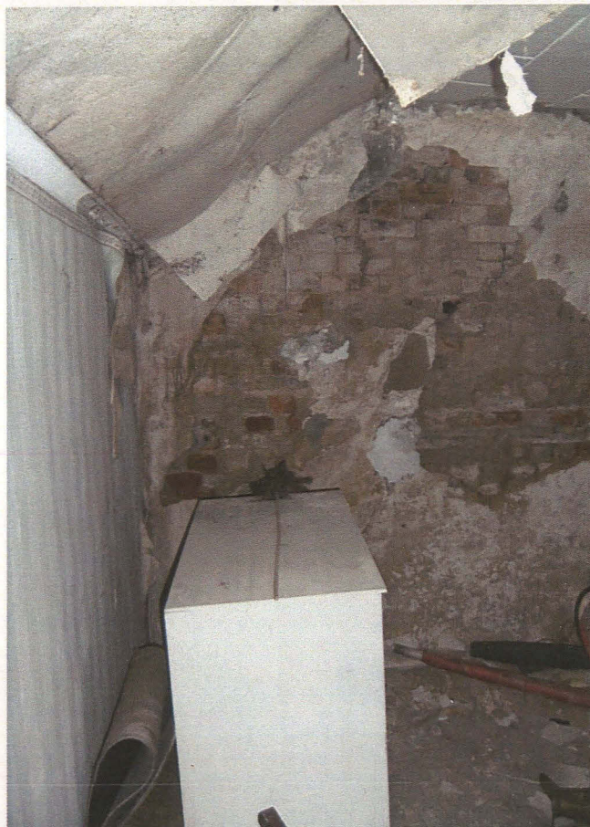
Plate 34 Interior of Room 1b, looking north
