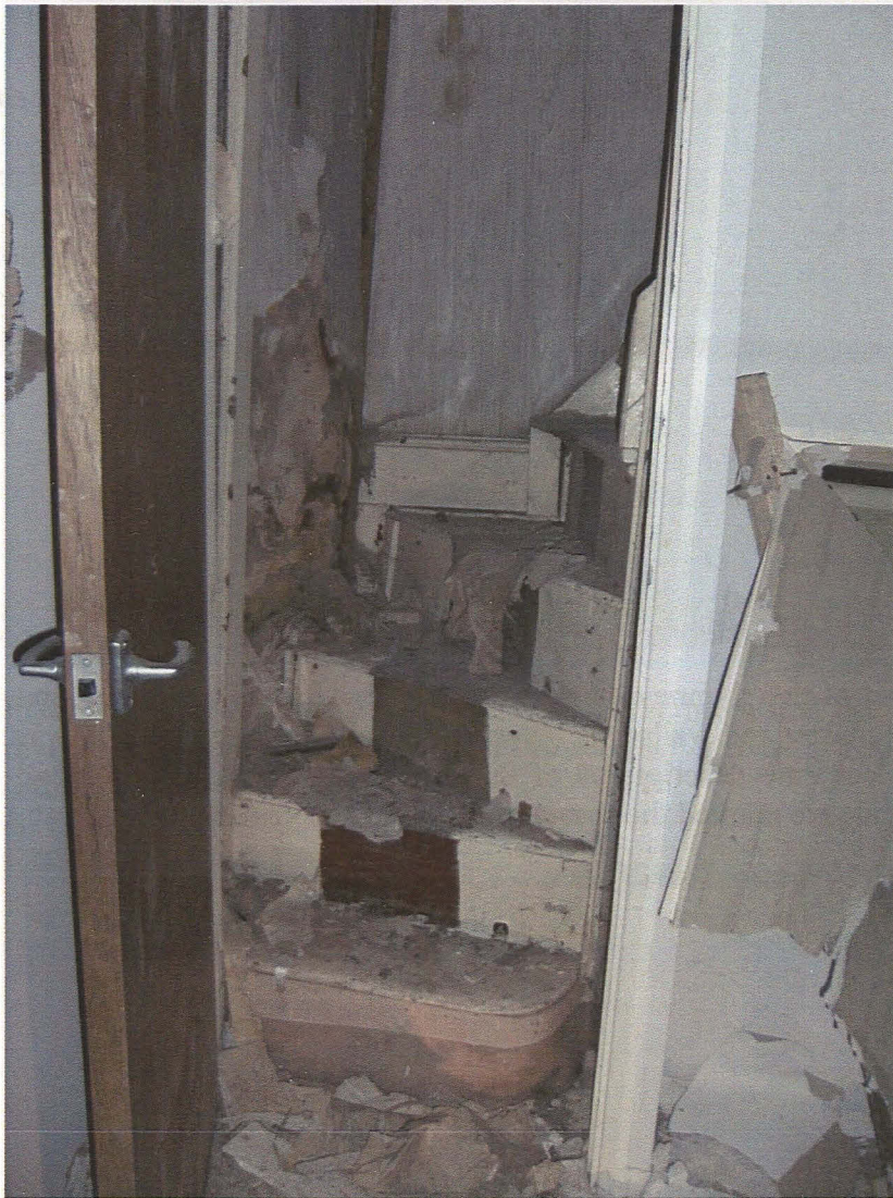
Plate 26 Interior of Room 1a, detail of staircase, looking south
