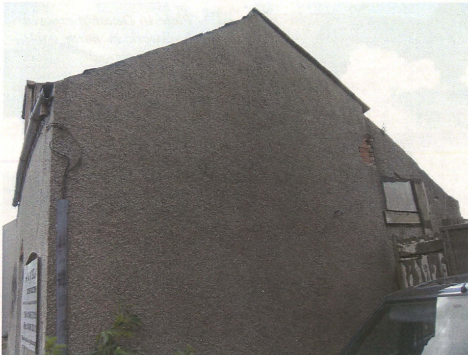
Plate 14 North gable end viewed from South Street, looking southwest
