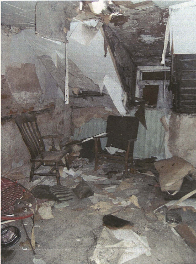
Plate 37 interior of Room 1a showing dormer window, looking northeast
