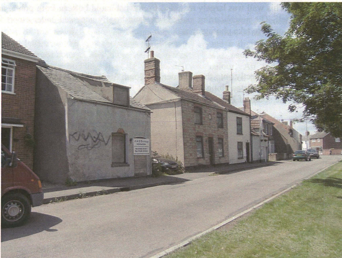
Plate 2 View of recorded building showing its setting in South Street, looking northwest
