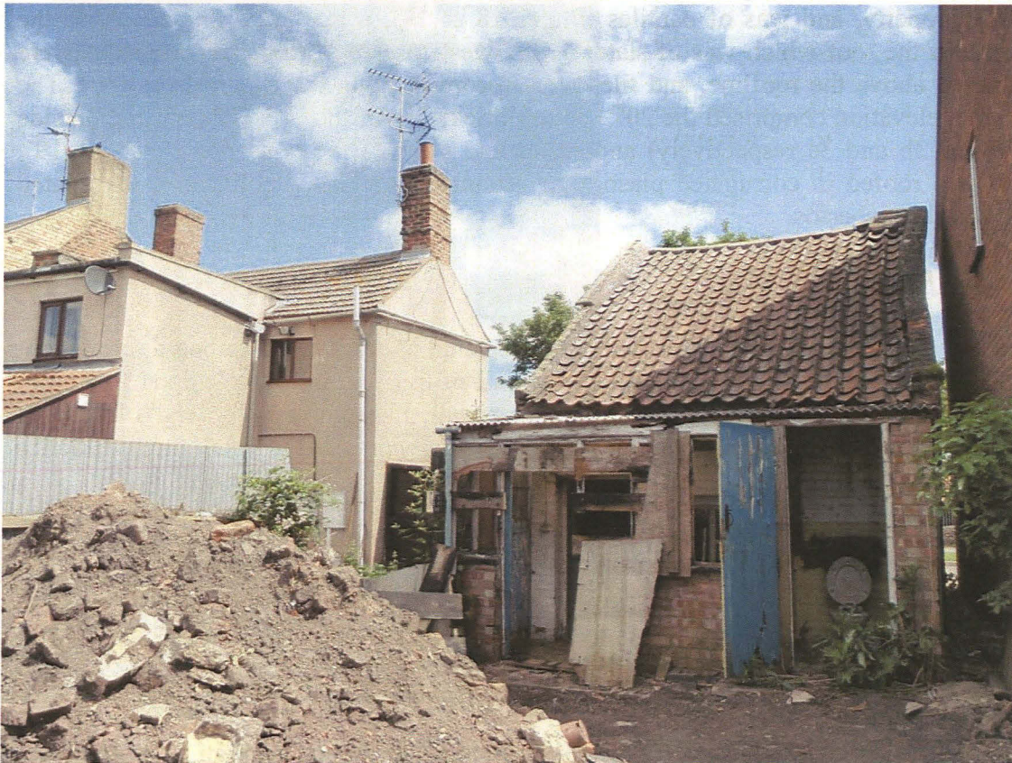
Plate 18 General view of west external elevation of cottage, looking northeast
