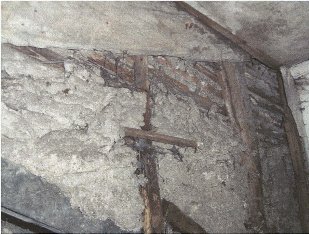
Plate 41 Interior of Room 1b, detail of laths and timber of north cheek of dormer window, looking northeast
