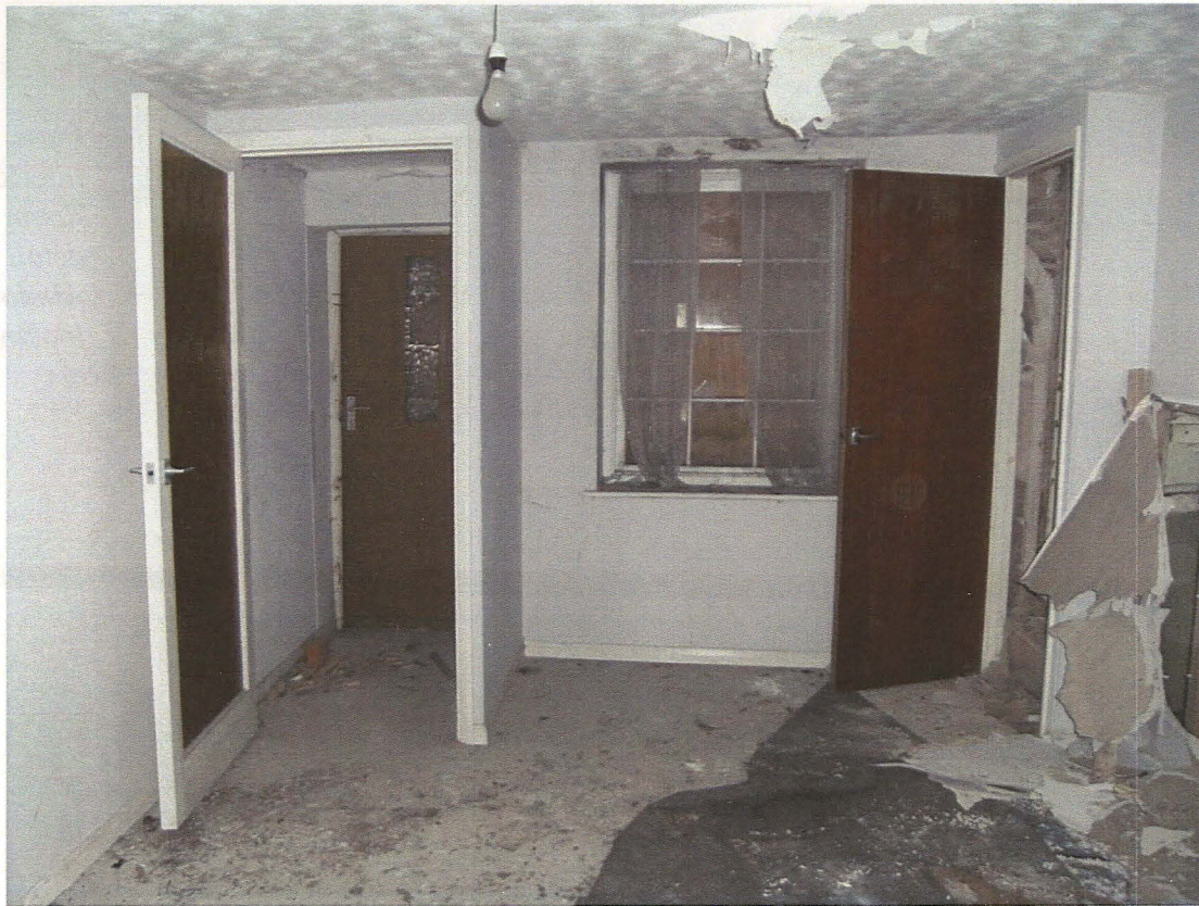
Plate 20 Interior of Room 1a, looking east
