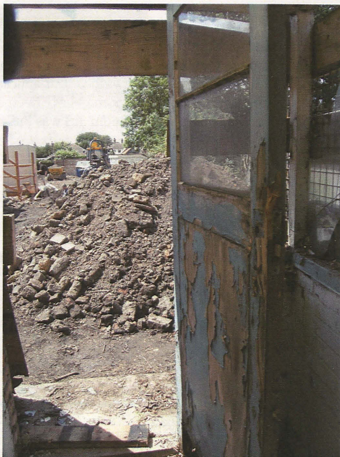
Plate 59 Interior of Room 2a, looking west to rear of property
