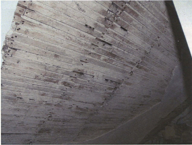
Plate 50 Interior of Room 2b, showing laths of ceiling, looking northwest
