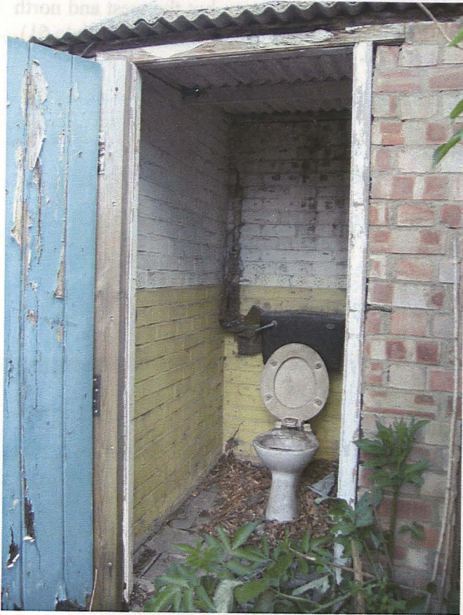
Plate 62 Interior of Room 3a, looking northeast
