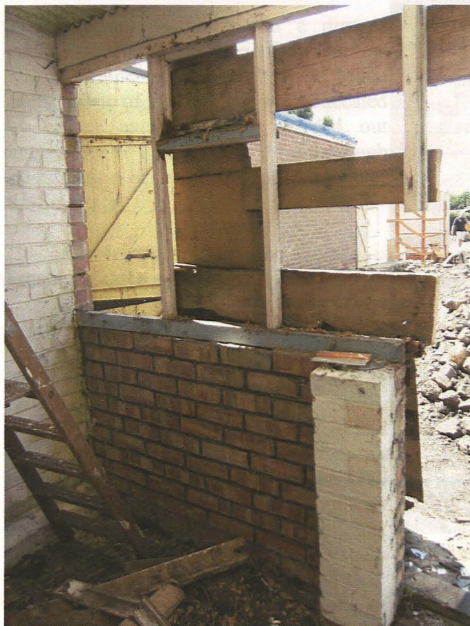
Plate 61 Interior of Room 3b, looking southwest
