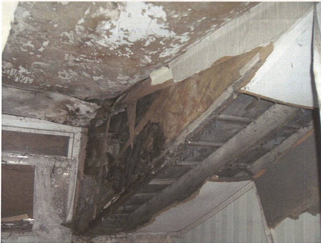
Plate 42 Interior of Room 1b, south cheek of dormer window, looking southeast
