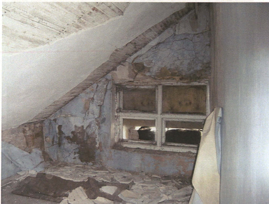
Plate 49 Interior of Room 2b, looking north
