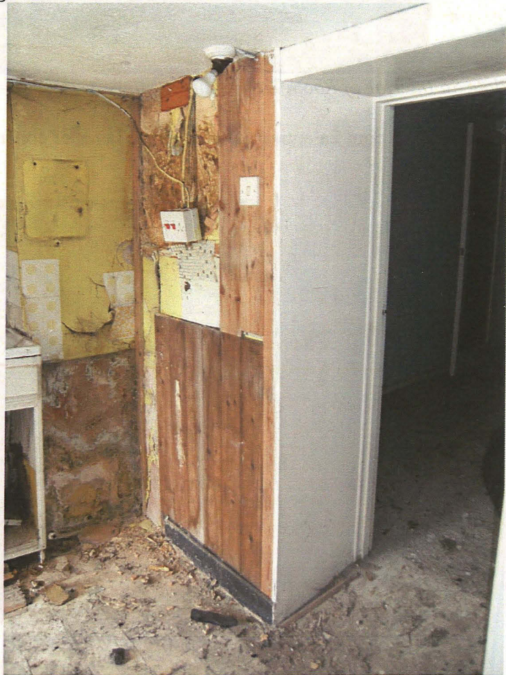
Plate 55 Interior of Room 2a, looking northeast
