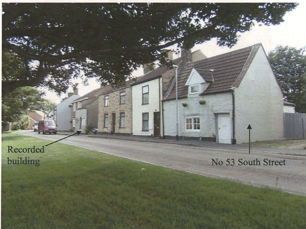
Plate 4 View along South Street showing recorded building and comparable cottage at 53 South Street, looking southwest
