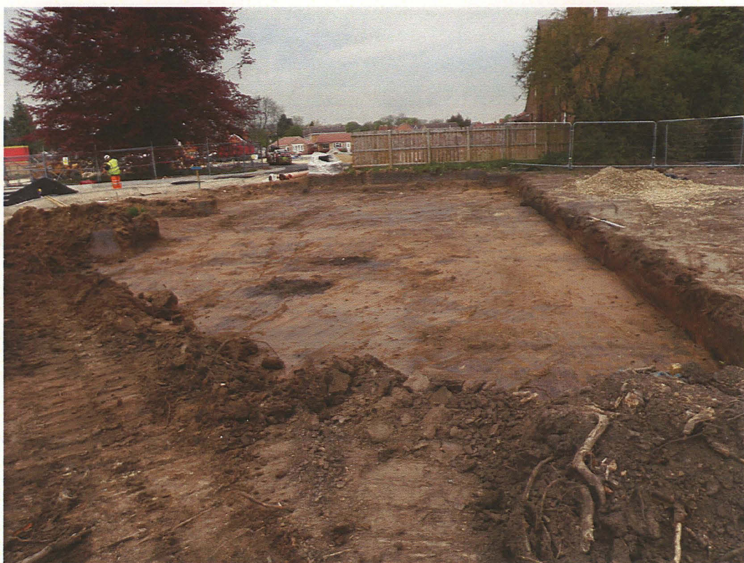
Plate 3. General view of southeast stripped area looking north
