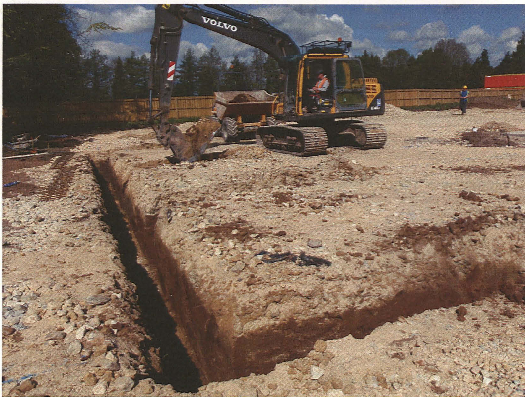
Plate 5. Machining of footings of Plots 18-20 looking west
