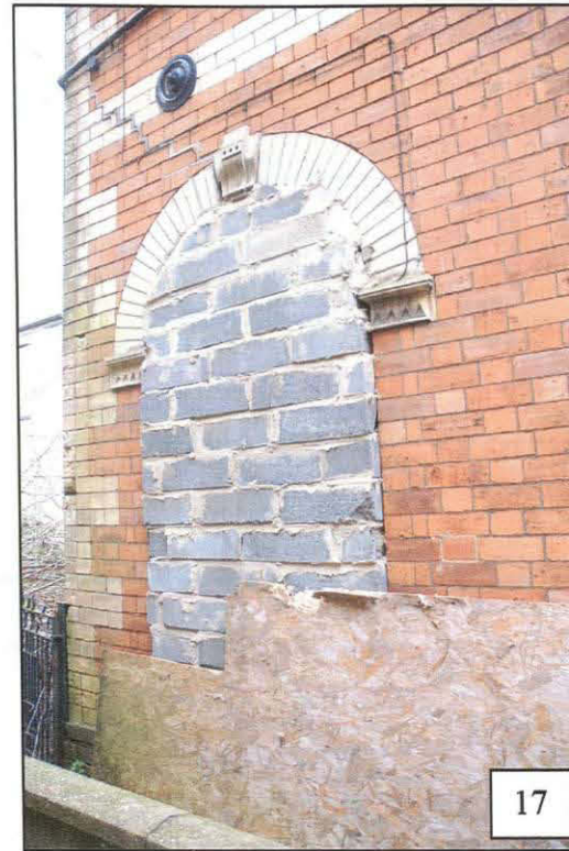
Plate 16: 47, St Catherines – Phase II blocked main entrance.
