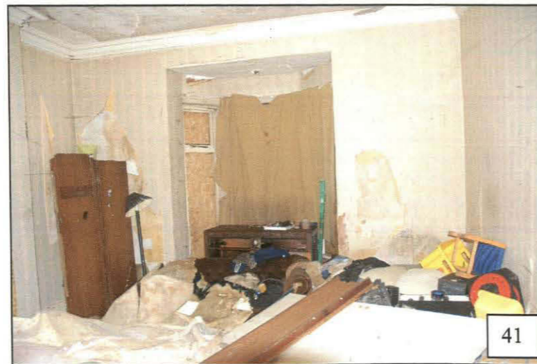
Plate 42: 47, St Catherines – Room 1, general view towards the main entrance.
