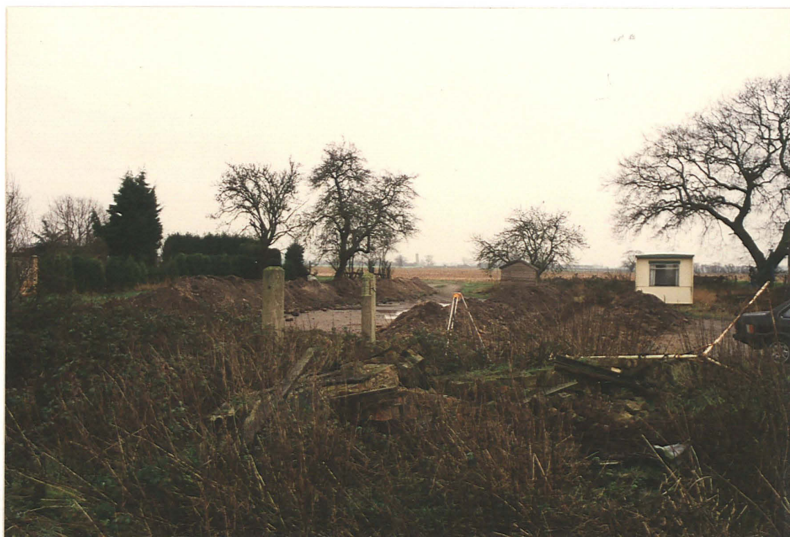
PI. 2 Development area with Trenches 1 and 2 opened. Looking SE towards fields containing cropmarks.
