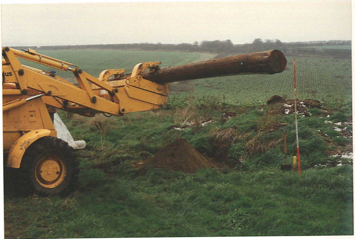
Pl. 2 Location of Pole 1 (looking SE)
