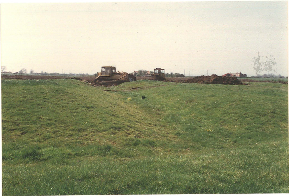
Pl. 4 Levelling of earthworks in progress, view looking west
