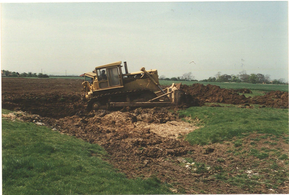
Pl. 5 Levelling of earthworks in progress, close-up
