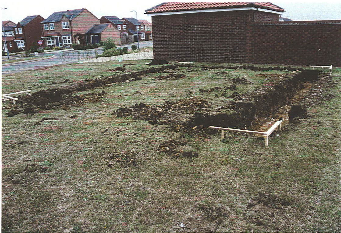
Photo. 4 General view of garage/showroom foundation trenches, looking north-east
