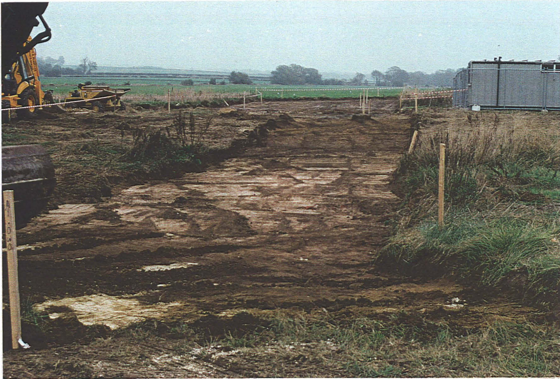
Pl. 1. Topsoil stripping of the new estate road (looking east).
