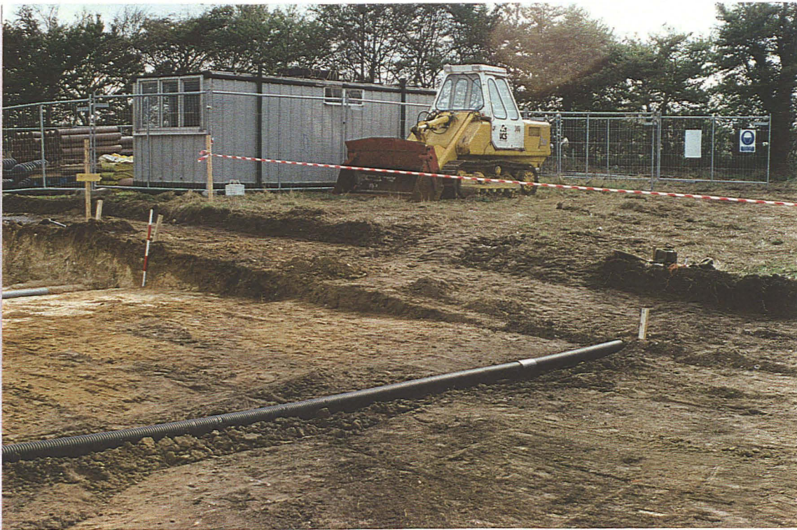
Pl. 5. Section through the upper fills of Ditch 100. The 1m scale marks a land drain cut (looking SE).
