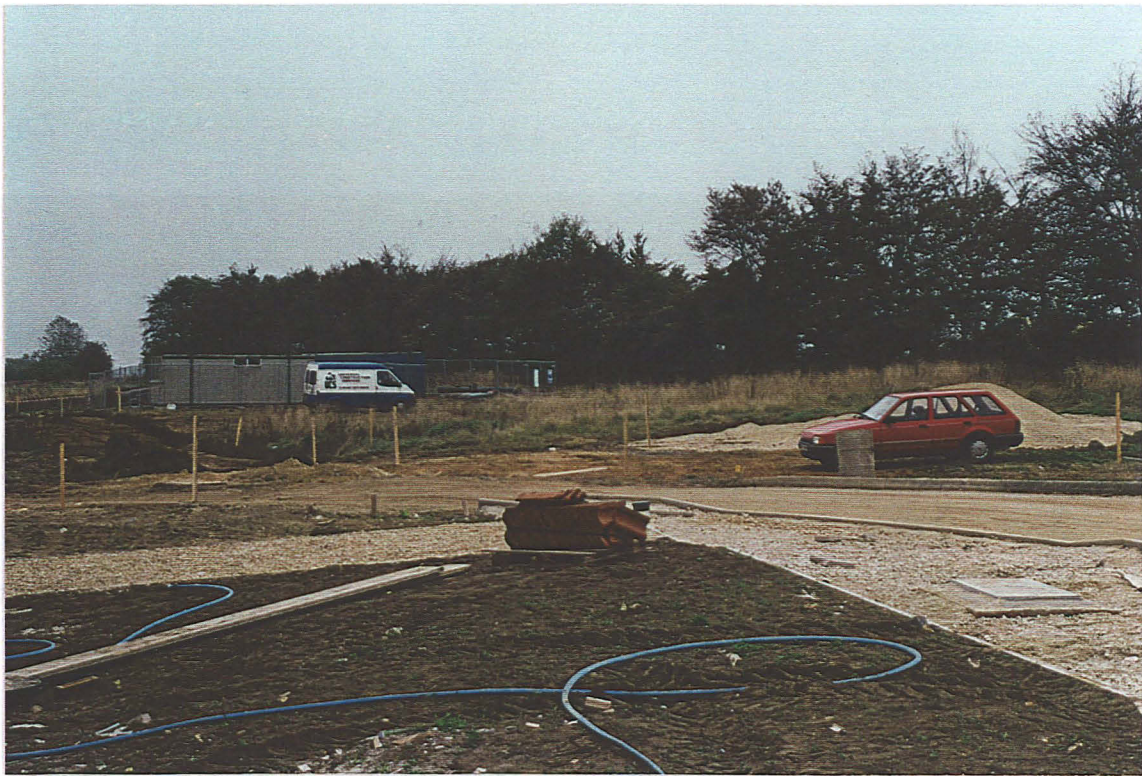
Pl. 7. The ridge visible as a marked feature in the field surface (looking SE).
