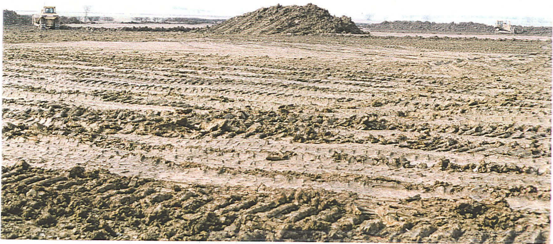
Plate 5: Main site area: top soil stripping
