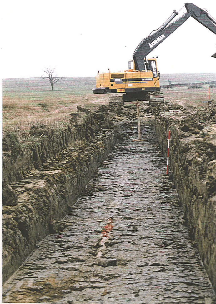
Plate 2: Access road cutting, looking south
