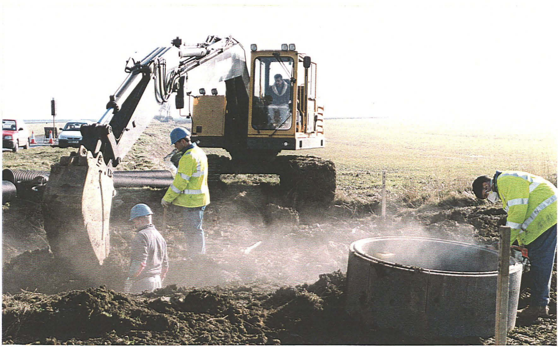
Plate 1: Excavation of manhole adjacent to B 1205, looking east
