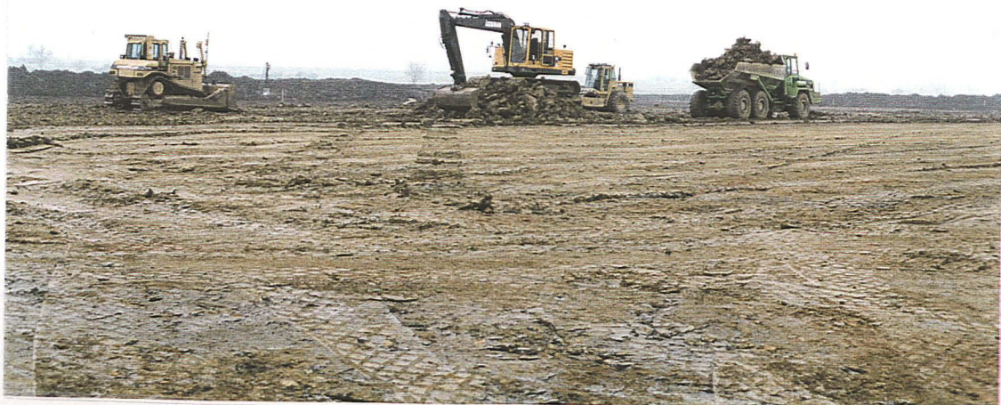
Plate 6: Main site area: 'cut and fill' operation
