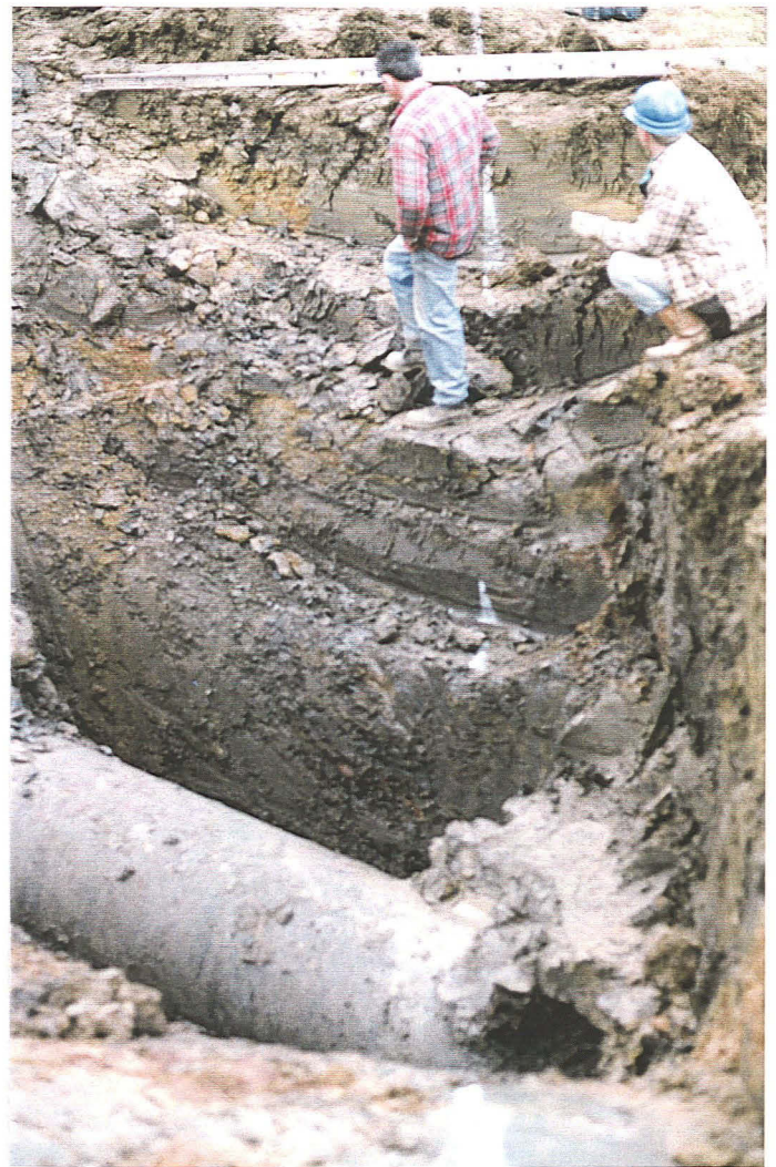
Plate 3: Inspection of 36" Gas Main crossing under access road, looking south
