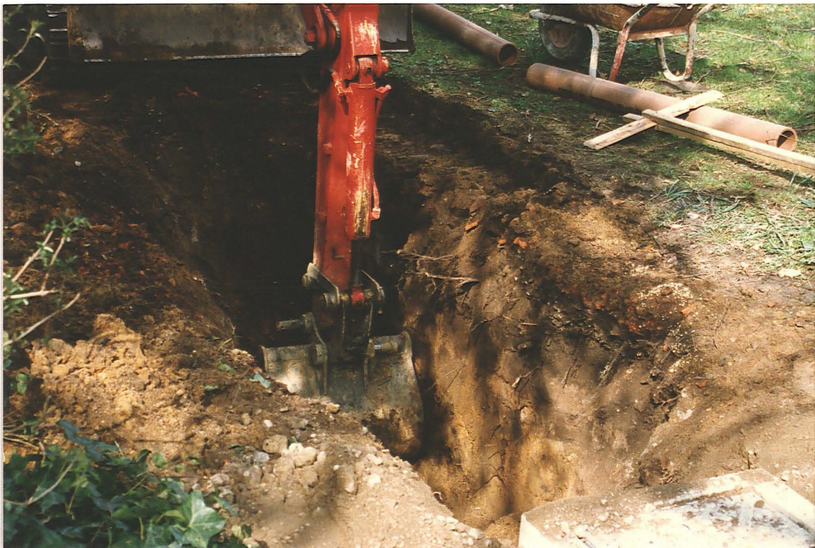
PI. 3 Rubble of the church path overlying the former topsoil above yellow undisturbed sand.
