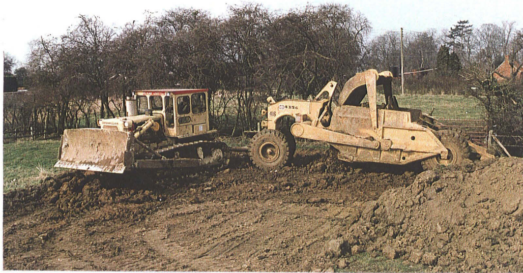
P3- Box-scraper dropping clay core in Flood Bank 2, looking north
