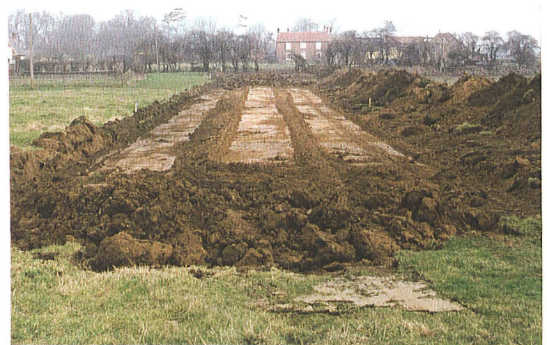
P4- Area stripped for Flood Bank 2, looking north
