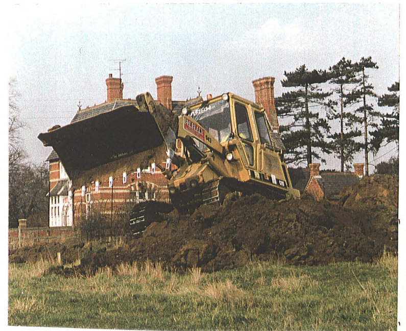
P8- Bulldozer working in Flood Bank 2, looking west
