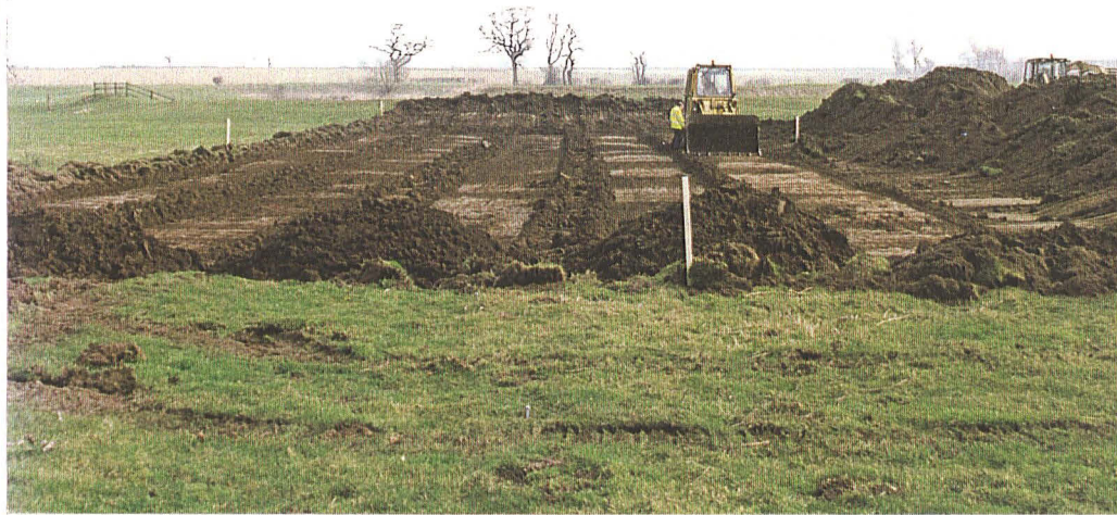
P1- Bulldozer scraping subsoil in Flood Bank 3, looking east
