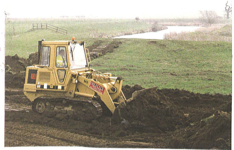
P6- Bulldozer stripping topsoil in Flood Bank 3, looking east
