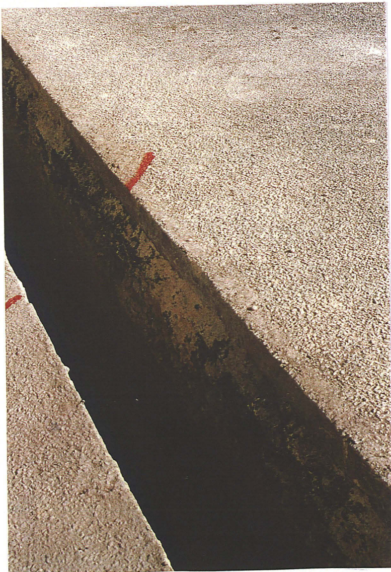
Pl. 7 Change from soil to dense rock at the eastern edge of 1 (marked by paint). Looking west.
