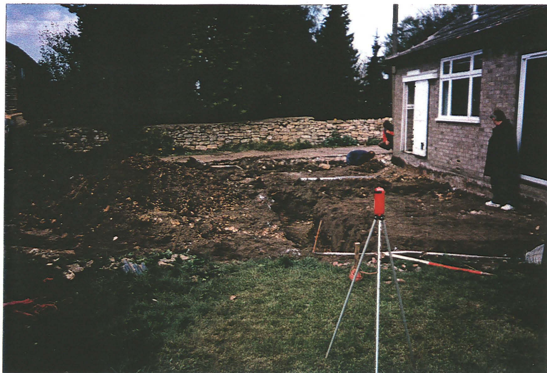
Plate. 1 General view of the foundation trenches for the extension, looking north.
