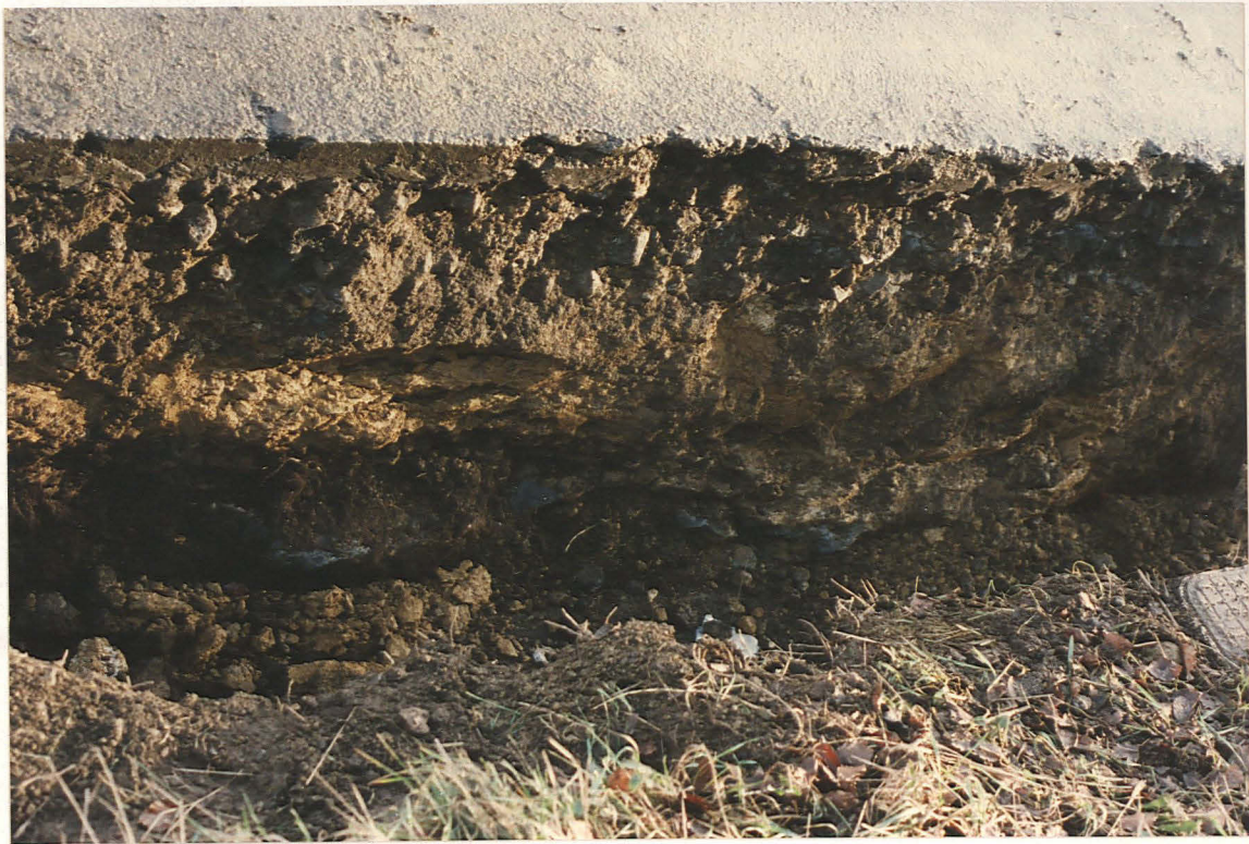
PI. 3 South of the Burton junction, the modern road had been built onto bedrock.
