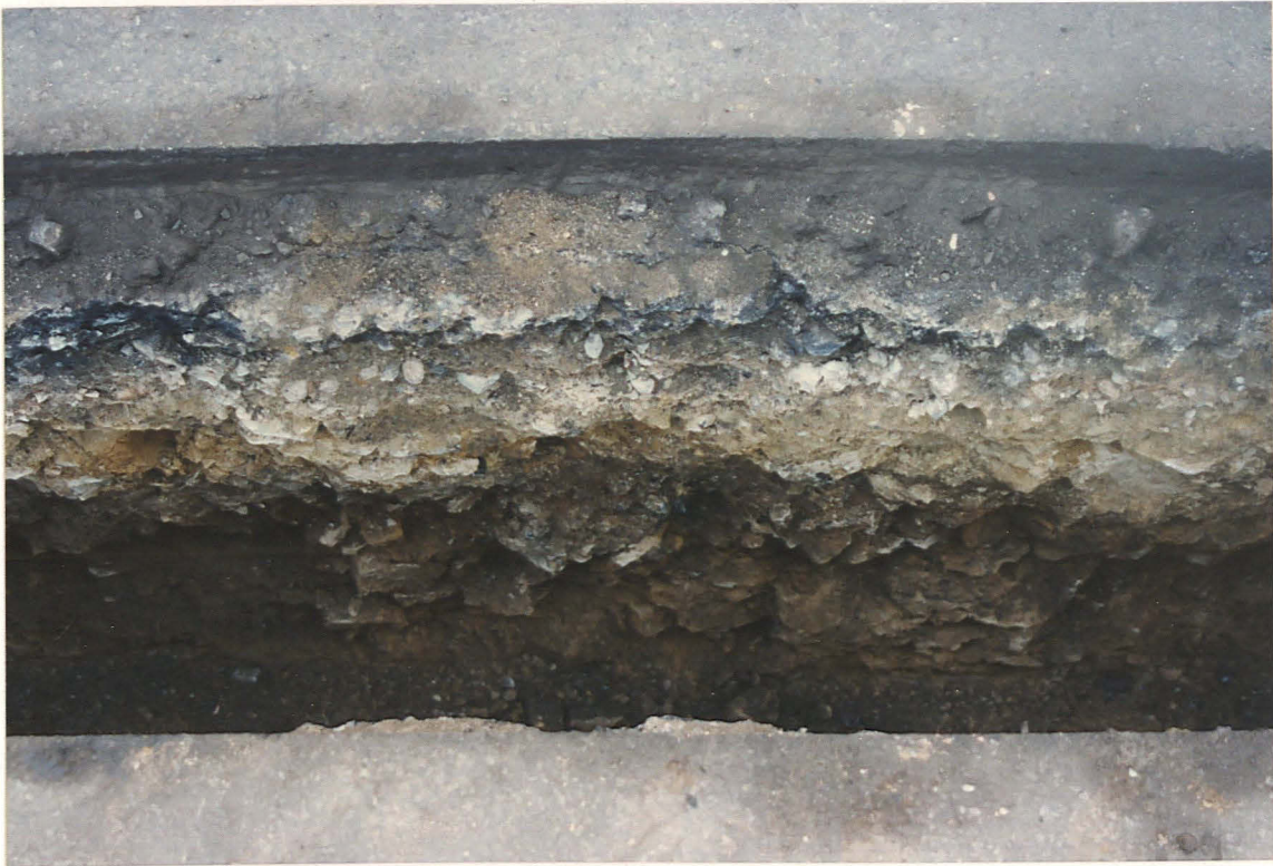
PI. 6 Road construction layers at the junction with Queen Elizabeth Way (8).
