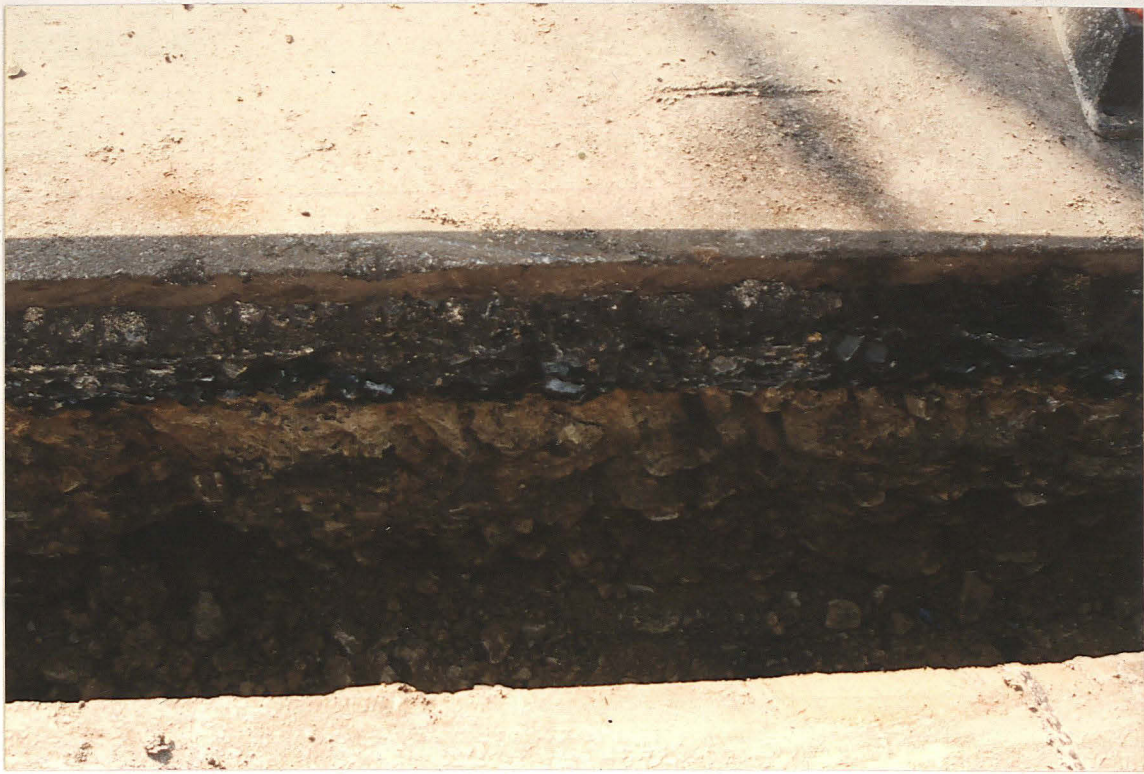
Pl. 7 Pitched limestone pieces close to Lincoln Lodge (9), thought to be the post-medieval road foundation.
