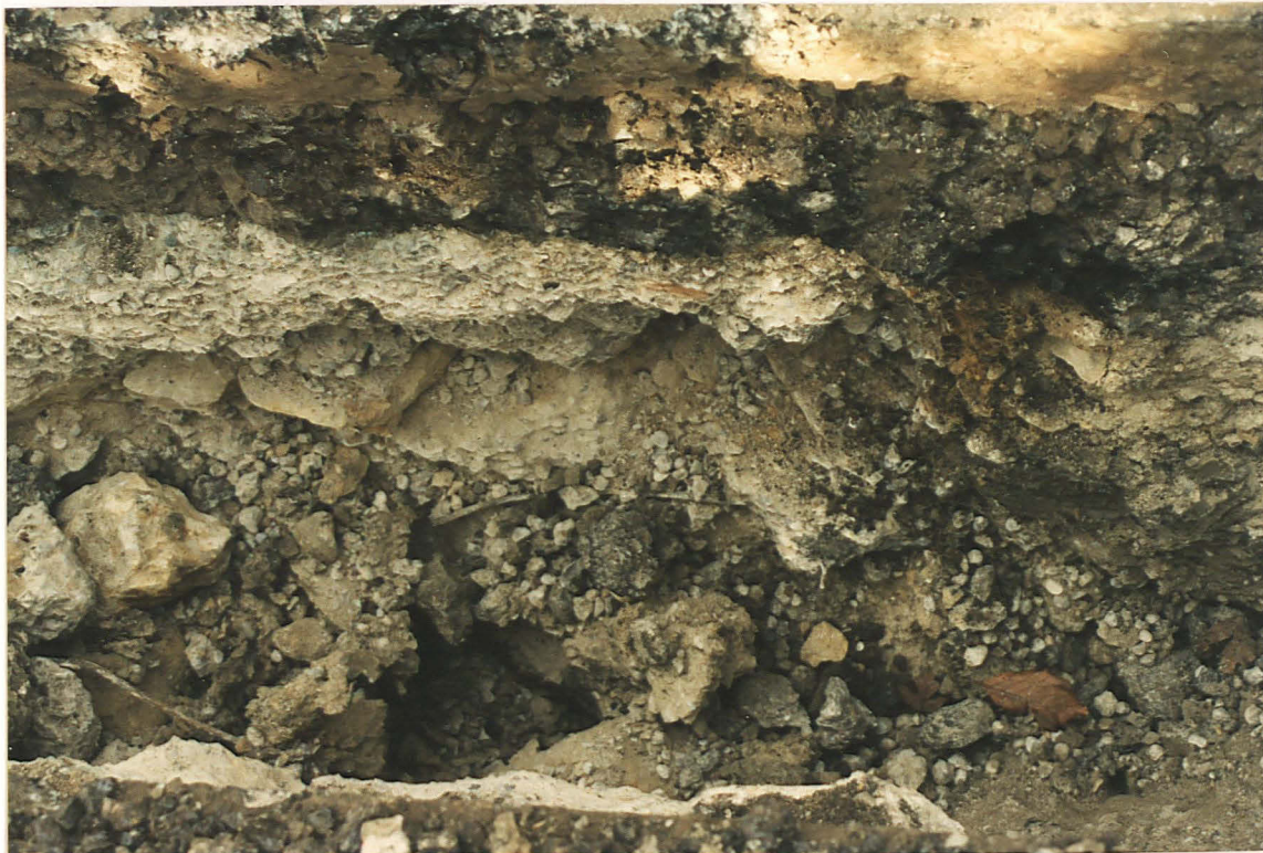
Pl. 2 Thick tarmac overlay concrete and stone to the west of the Middle Street/Burton Main Street junction, probably serving to raise the road level.
