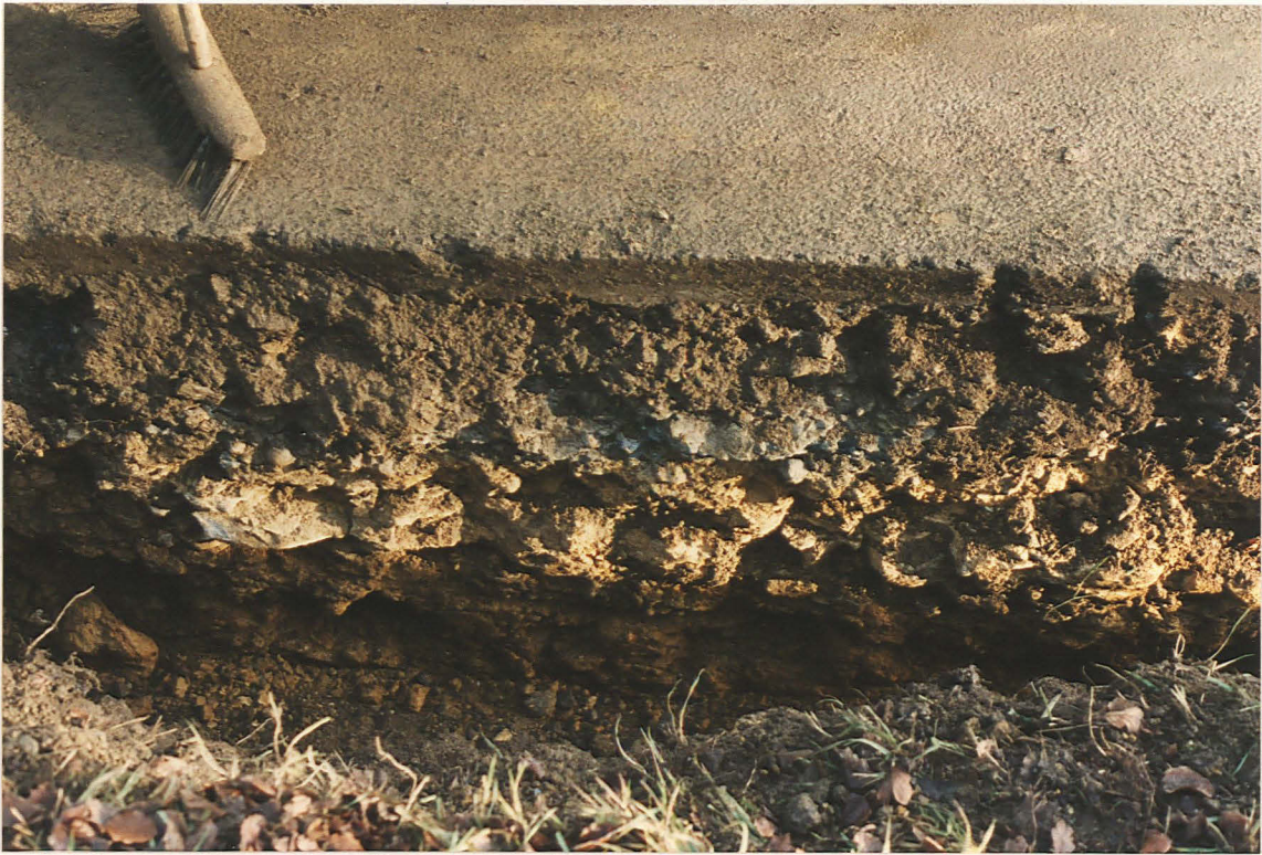
PI. 5 Mixed layers of road construction material; at 3 the lowest visible layer may have been weathered bedrock, suggesting that little or no truncation of deposits had occurred.
