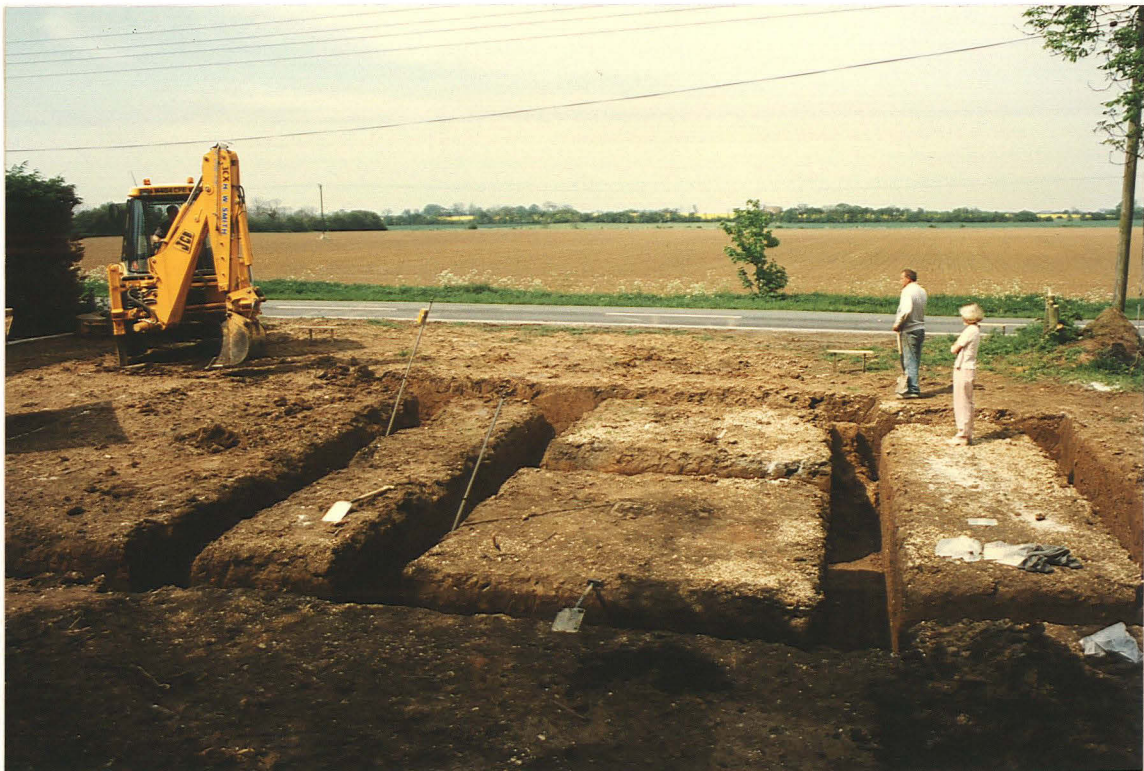
PI. 6 Foundation trenches from south.
