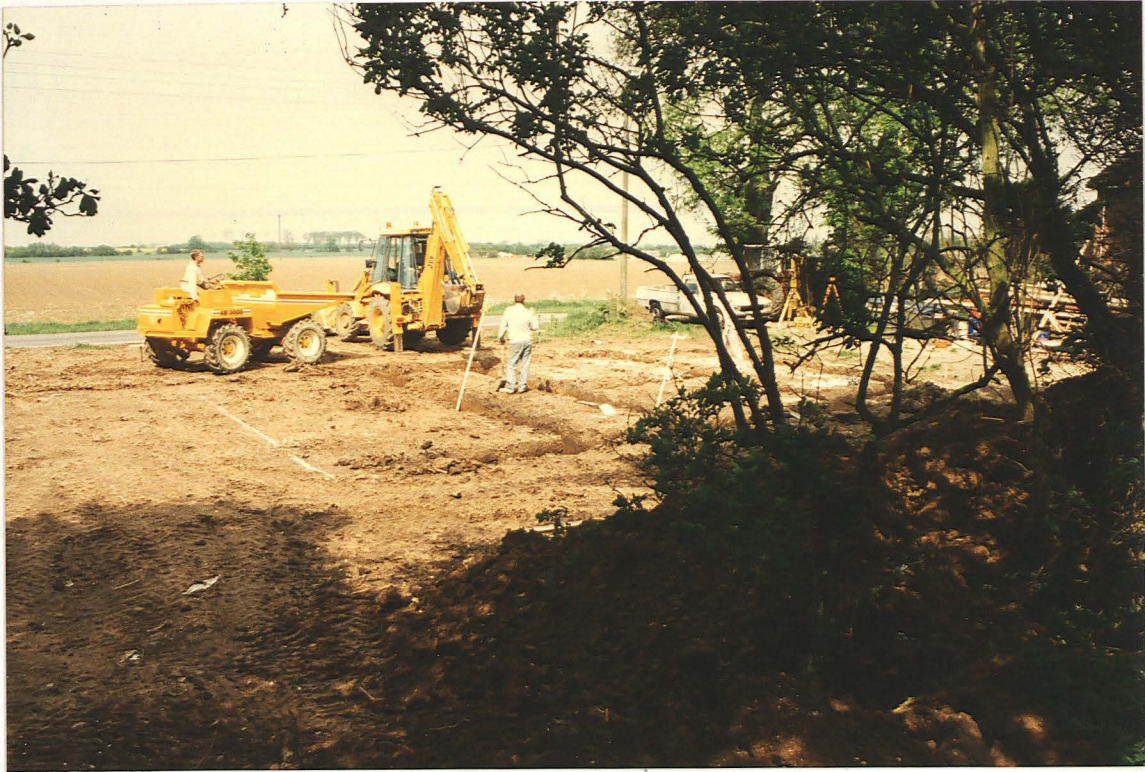
PI. 5 Foundation trenches from SSW (moat bank).
