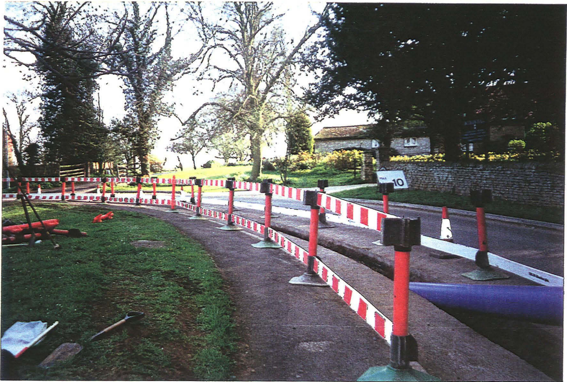
1. General view of pipe laying operations in Witham-on-the-Hill
