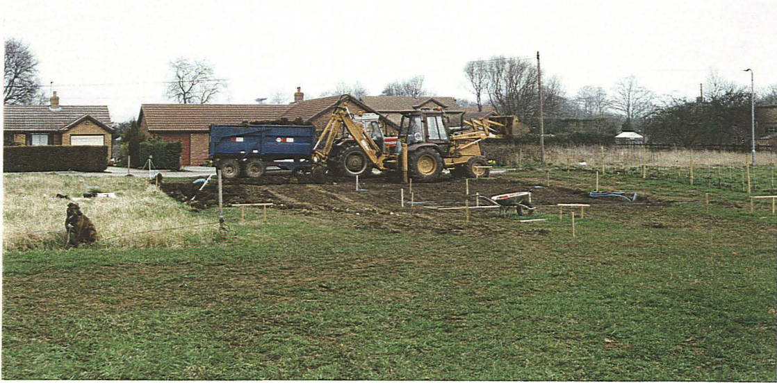
Photo. 1 General view of house foundation plot during trenching, looking north-west
