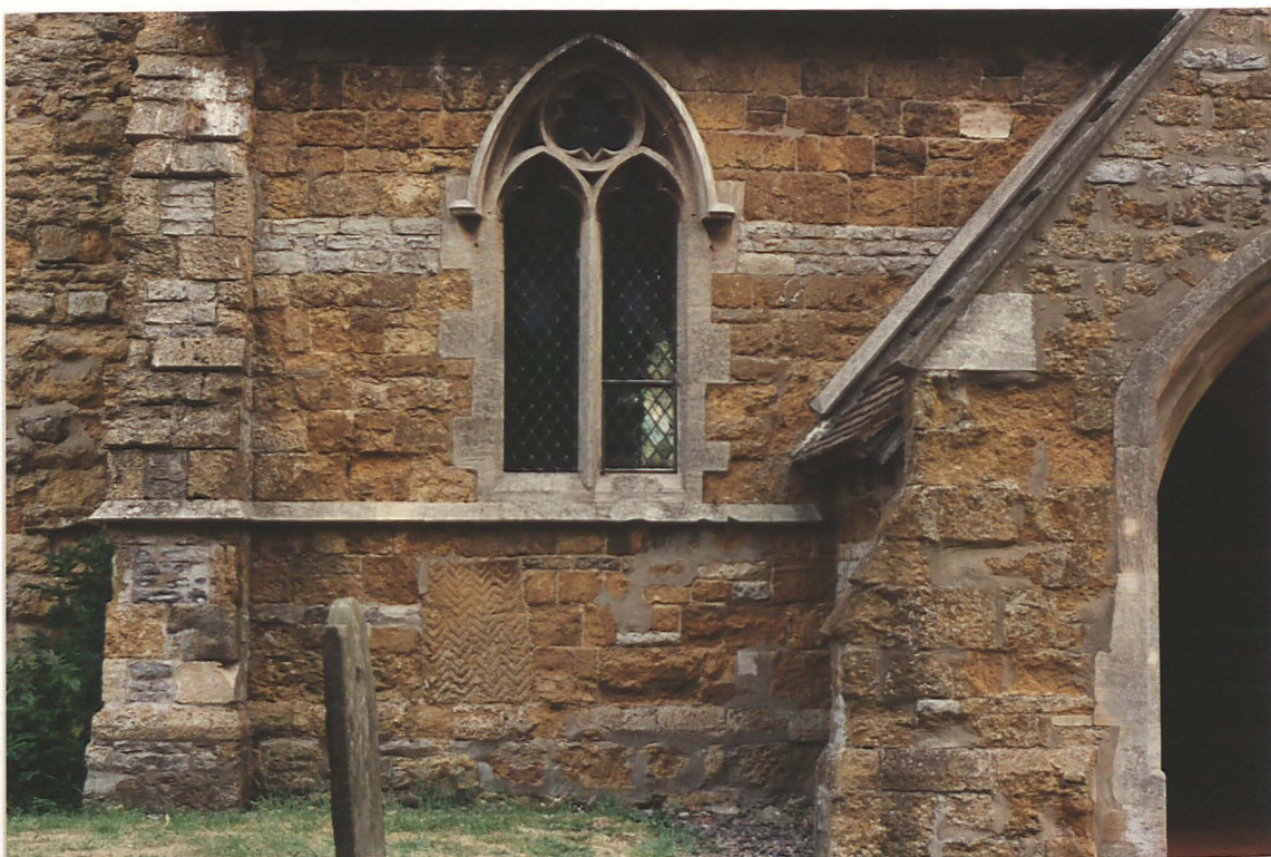
Pl. 9 Saxo-Norman decorated stone re-used in the nave south wall of North Kelsey Church (looking north)
