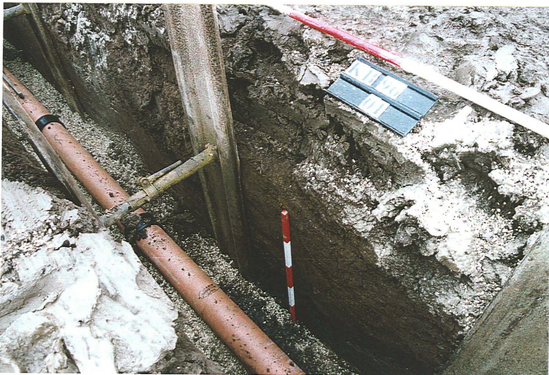
Ditch [01] exposed in east-west sewer trench, looking south-east
